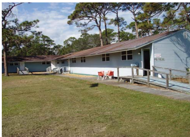
Figure 3-2. KARS Park recreation building.
