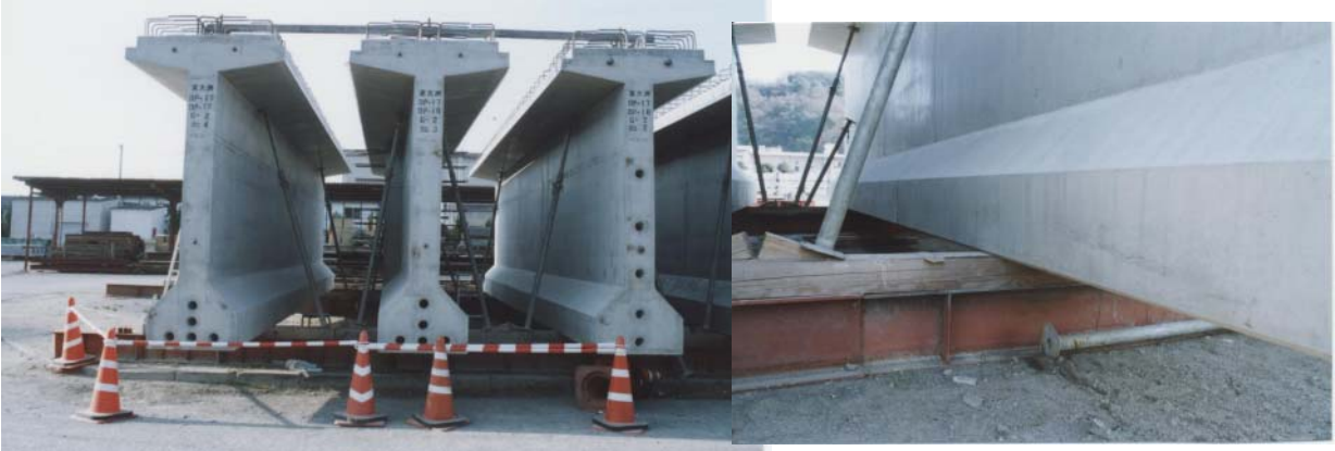
Photo 3 Condition of Concrete
