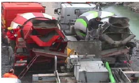
Fig. 8 Arrangement for continuous discharge
