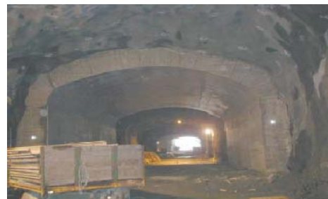
Fig. 9 View of the south arch
