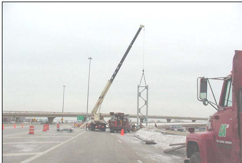
Figure 6. End Frame Being Set Onto Its Foundation.
