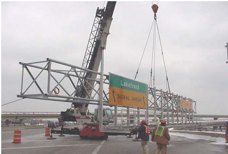
Figure 7. Assembled Truss Being Lifted Into Place.
