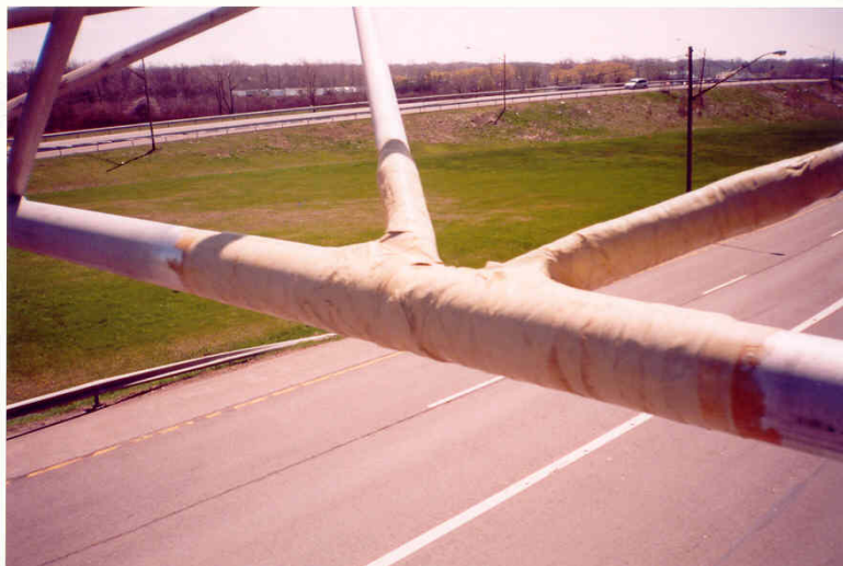
Figure 37. Repair of Truss Members Using FRP.
