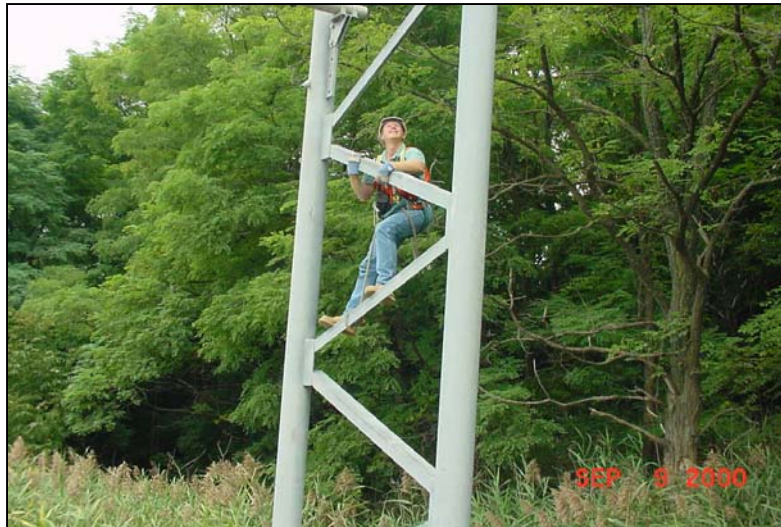
Figure 17. Inspector Climbing Structure.
