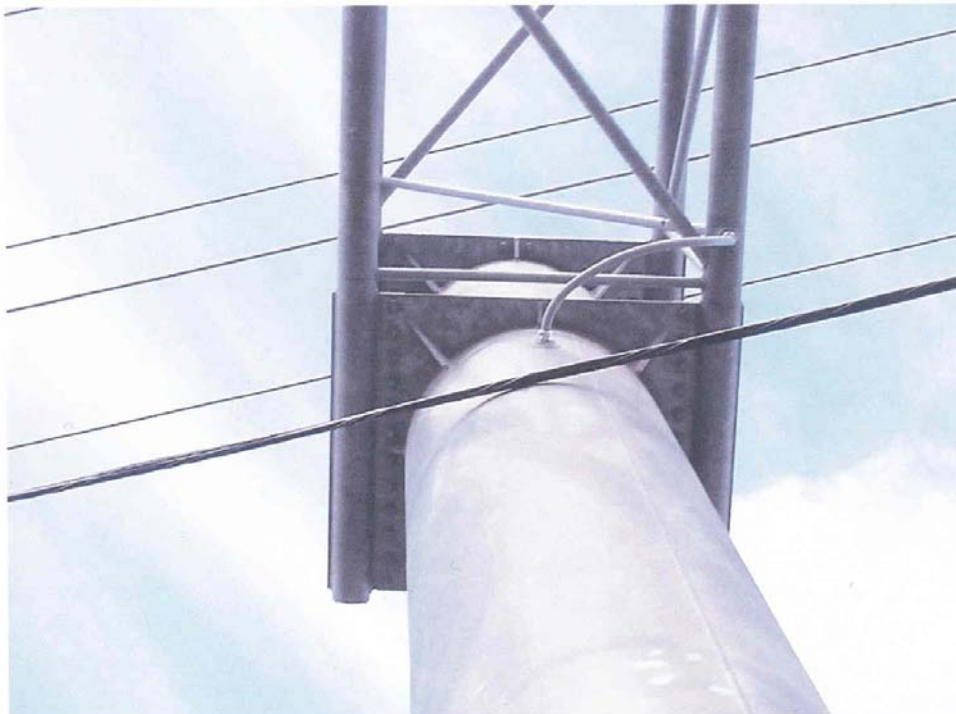
PHOTOGRAPH 4: COLUMN TO ARM CONNECTION
