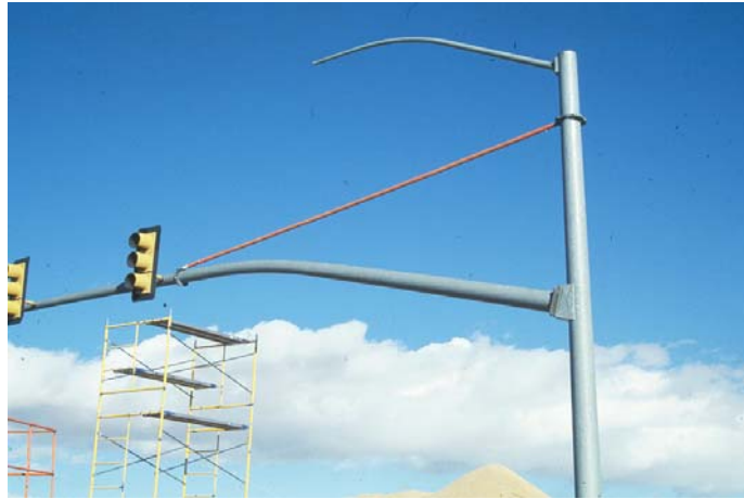
Figure 40. Wyoming Strand Damper.
