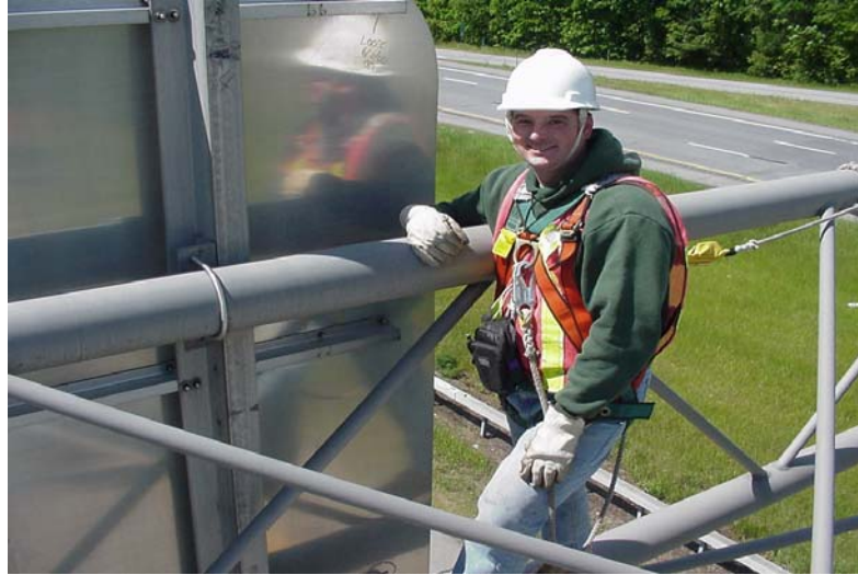
Figure 19. Inspector Uses Double Lanyard System.
