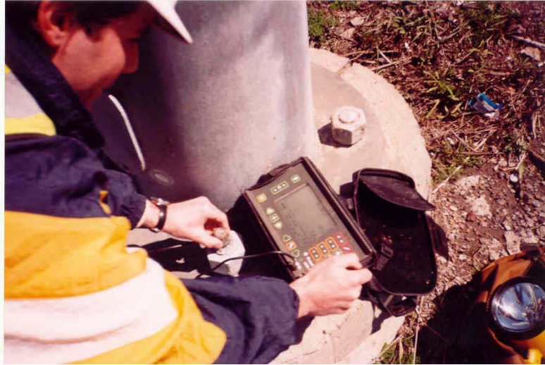
Figure 33. Ultrasonic Testing of Anchor Rods.
