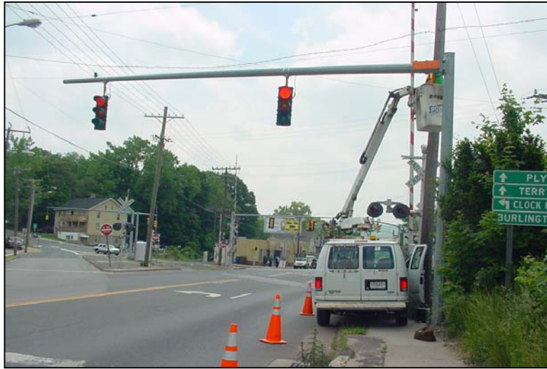
Figure 26. Inspection of a Mast Arm Structure.
