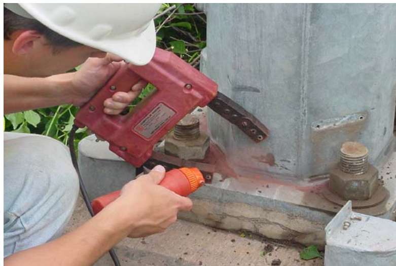
Figure 34. Magnetic Particle Inspection of Weld at Post to Base Plate Connection.
