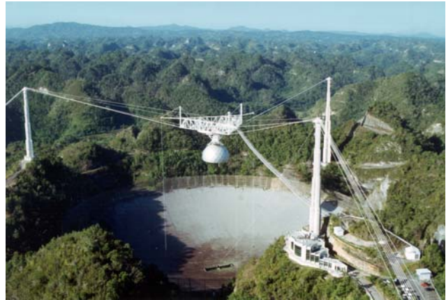
An image of the Arecibo Radio Telescope in Puerto Rico. The Gregorian dome and its suspension structure are visible over the main deflector below. Credit: Arecibo Observatory/NSF
