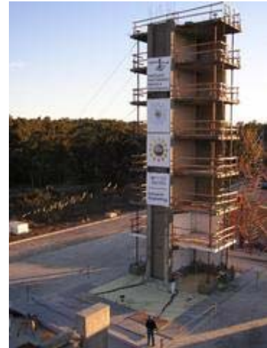
The seven-story, 275-ton reinforced concrete structure tested on the University of California, San Diego NEES shake table demonstrated a less costly seismic design method for residential structures in southern California. Credit: Professor Jose estrepo, Department of Structural Engineering, UCSD
