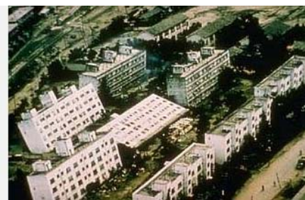
Entire buildings tilt because of ground failure after the Niigata, Japan, earthquake. Credit: NGDC.
