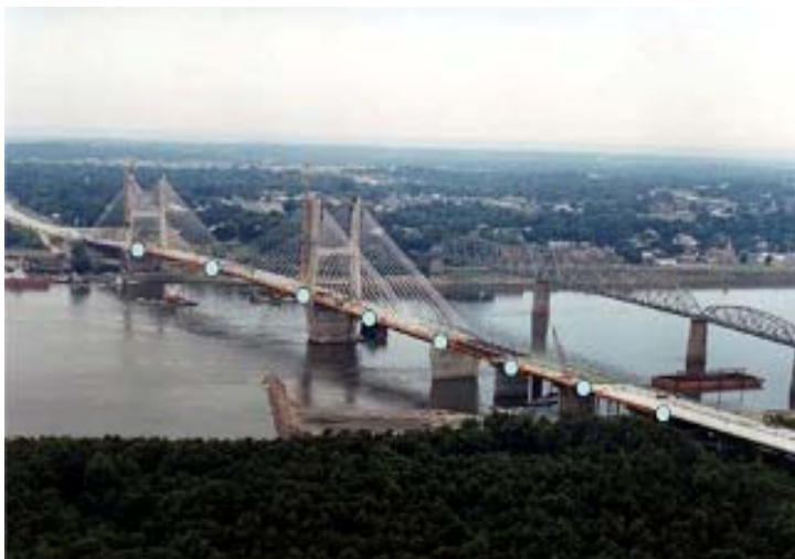
This picture shows the Bill Emerson Memorial Bridge in Cape Girardeau, Missouri, when it was under construction. It is the main crossing on the Mississippi River and lies in the New Madrid seismic zone. The real-time wireless sensor network system developed in this project is being deployed to insure the bridge's safety. Credit: Missouri Department of Transportation.
