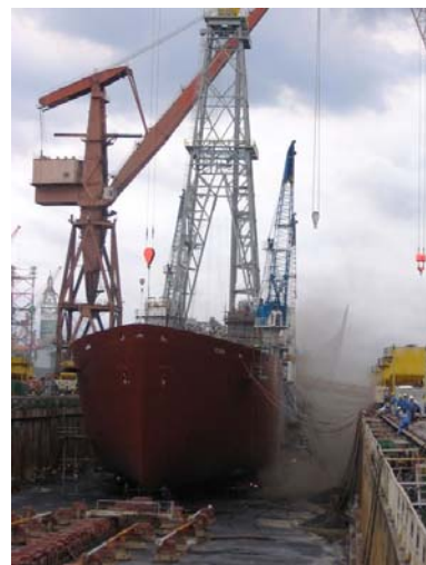
The Scientific Ocean Drilling Vessel JOIDES Resolution in drydock at the Jurong Shipyard in Singapore undergoes blasting and painting in July 2007. Credit: NSF.
