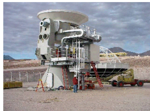
The first Vertex antenna under assembly at the ALMA site in Chile. Credit NRAO/AUI
