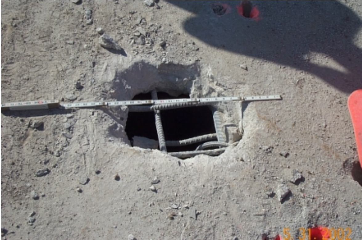
Attachment 13 – 18” Holes drilled into the Deck
