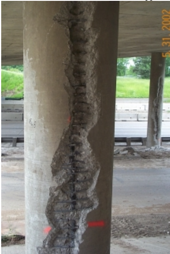
Attachment 14 - Columns Before Wrapped
