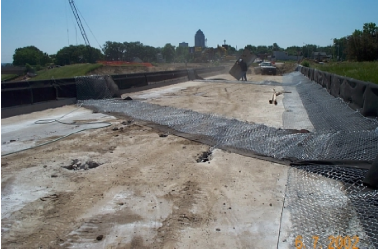
Attachment 11 – Deck Wrapped only over Pier Caps and Sidewalk
