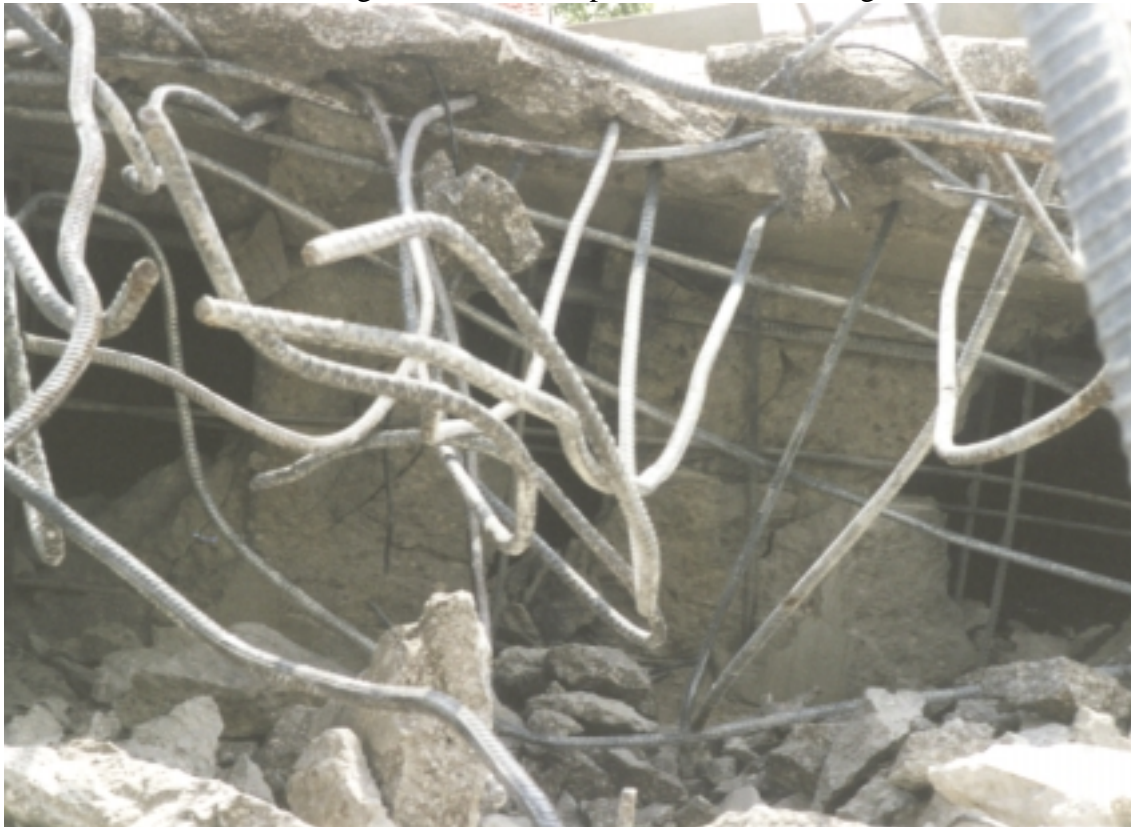
Attachment 17 – An inside girder after the implosion once outside girder was removed
