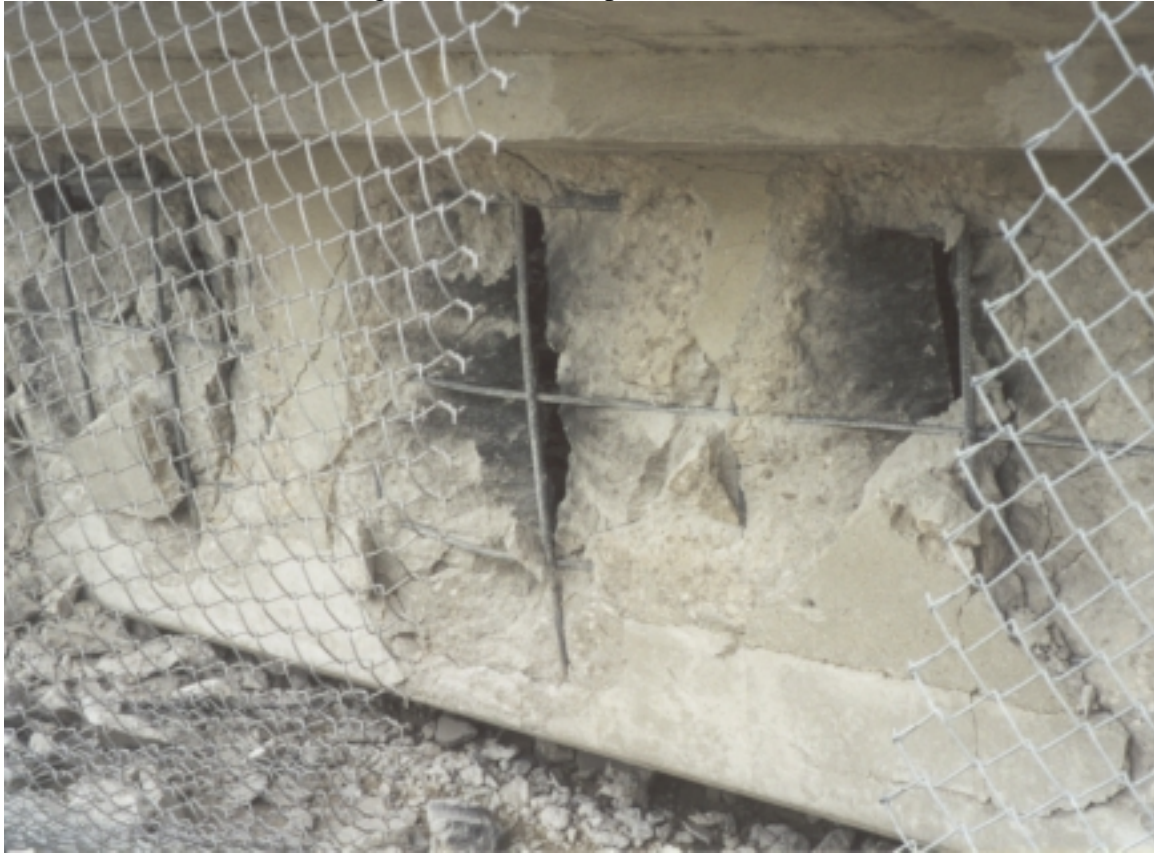
Attachment 16 – An outside girder after the implosion
