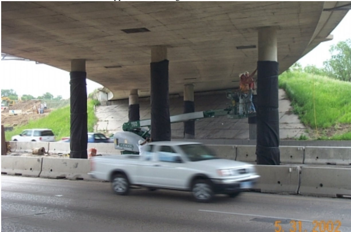
Attachment 10 – Columns wrapped with fencing and fabric
