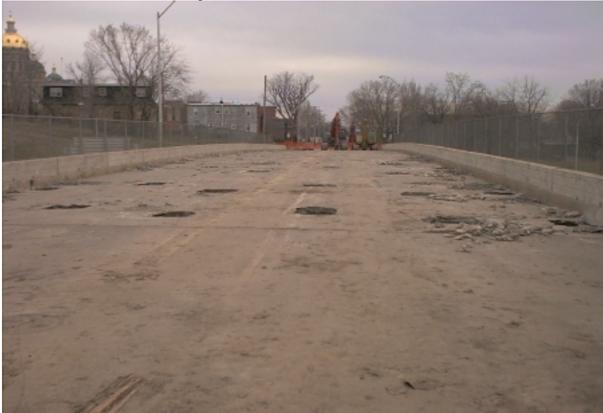
Attachment 1 – E 9 th – Evening Before Demolition
