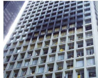
View of east side of the Cook County Administration building, Chicago, Illinois.
