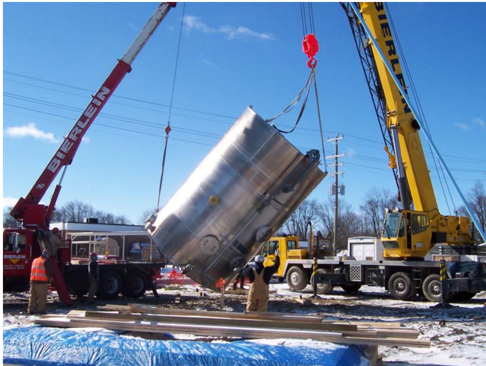
Figure 4-8. Equipment Delivery and Unloading
