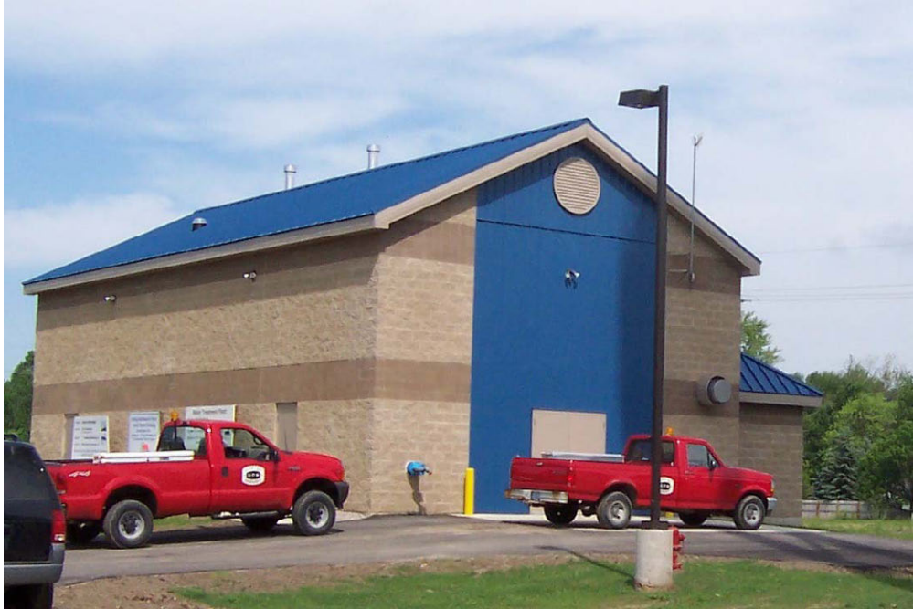
Figure 4-7. New Treatment Plant Building
