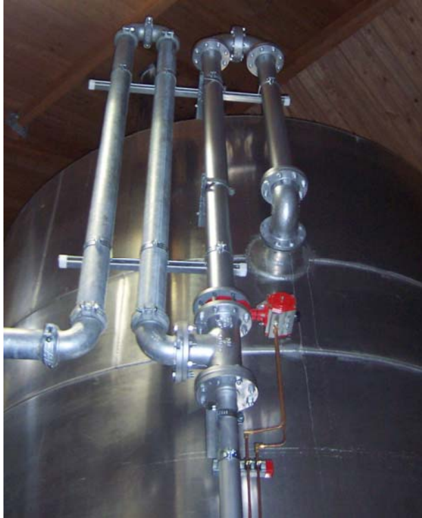
Figure 4-9. Blower Piping Modification
