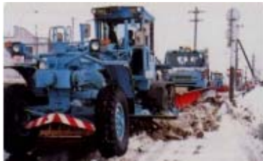
snow removal on roadways
