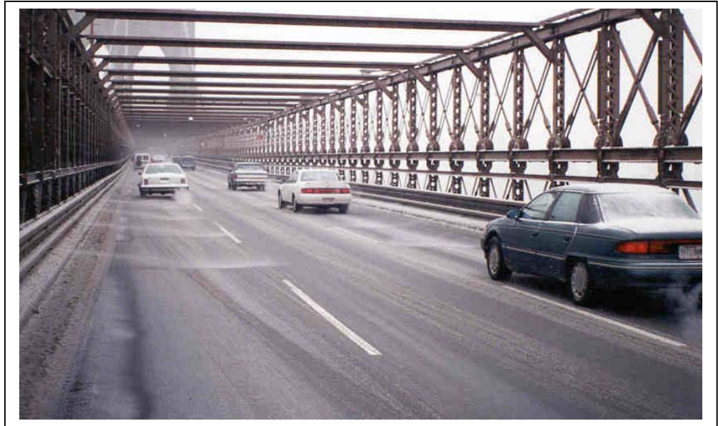
Photo Exhibit H: FAST system spraying (1/14/99)
