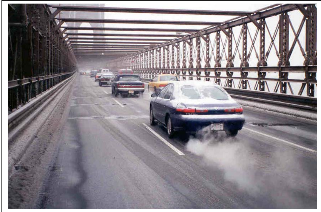
Photo Exhibit D: Pavement condition before re-treating (1/14/99)
