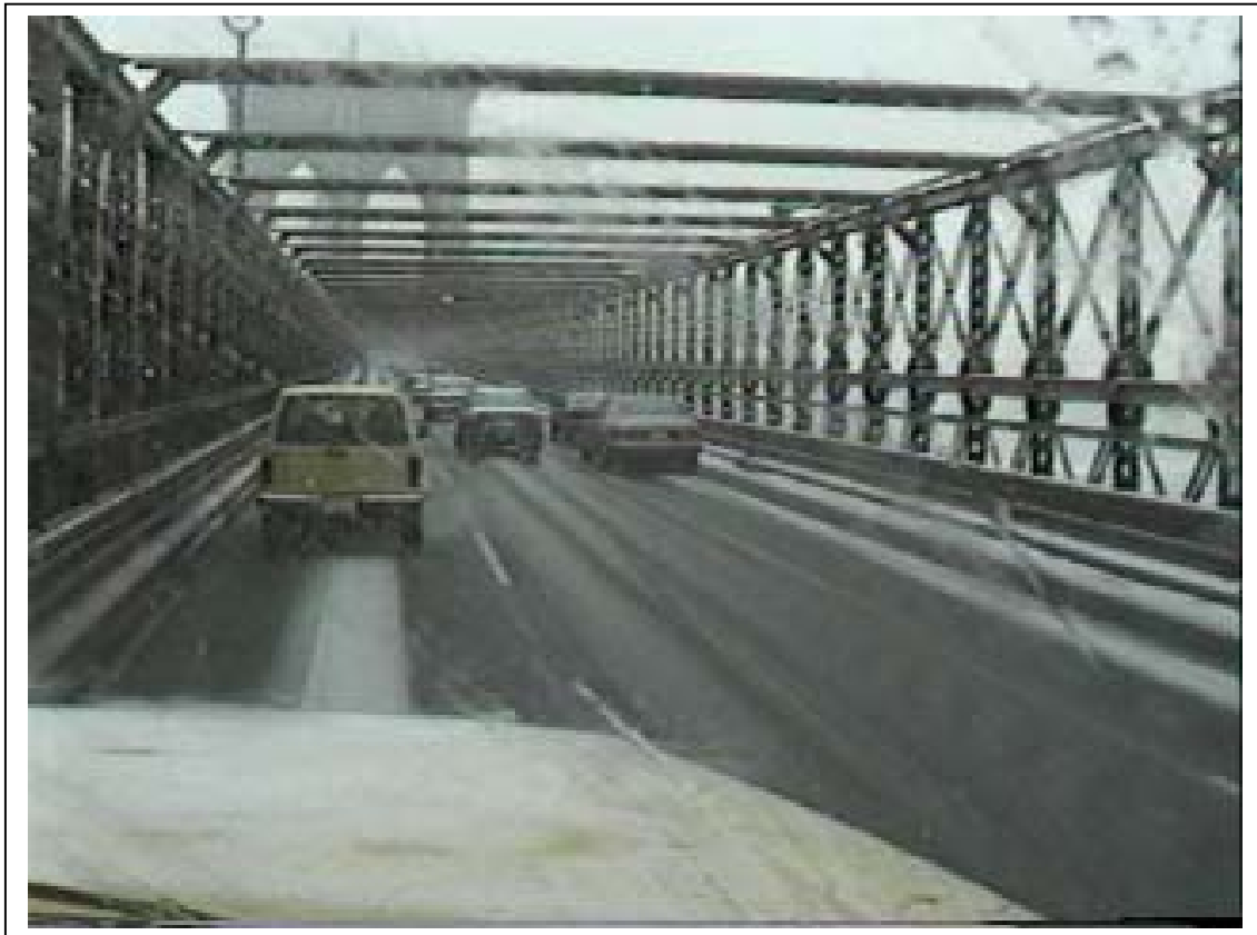
Photo Exhibit A: Pavement condition of roadway section sprayed with FAST system (3/14/99)
