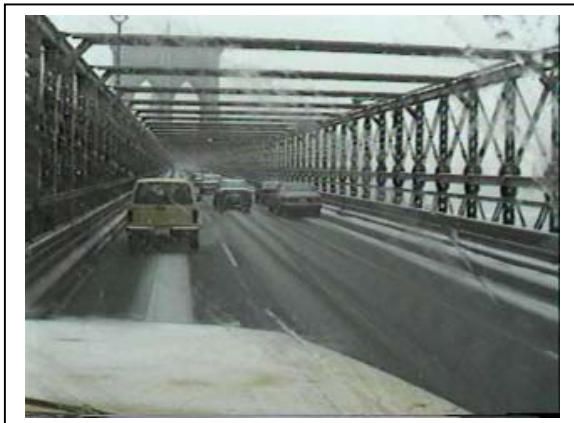
Photo 1: Road section sprayed by the FAST system
