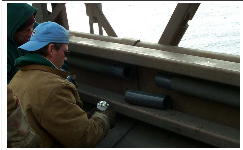
Photo Exhibit J: Typical joint repair
