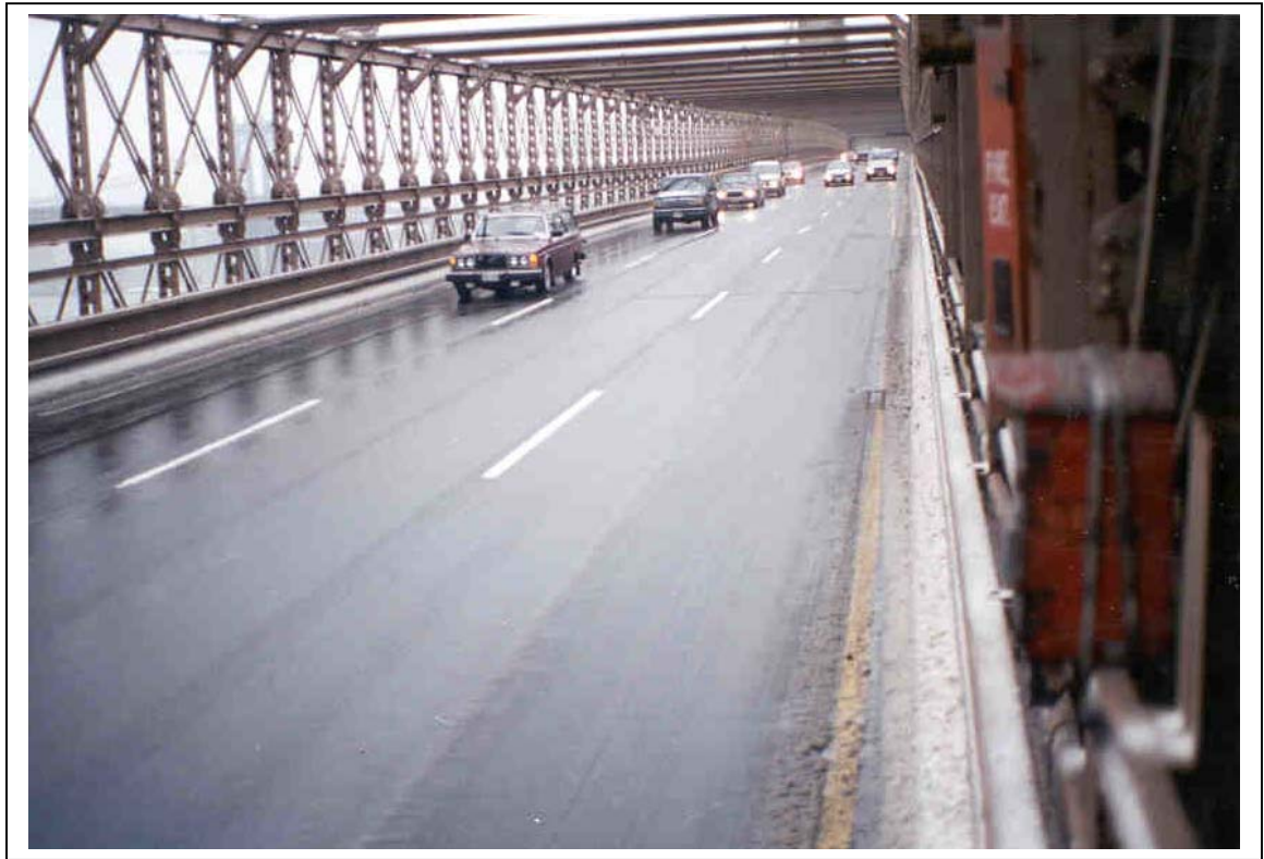
Photo Exhibit F: North roadway pavement after >4 passes of DOS salt trucks (1/14/99)
