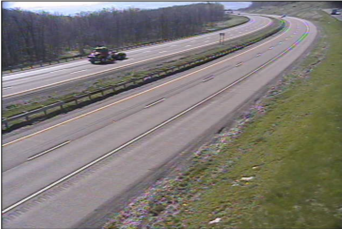
Figure 4. Daytime view from the RWIS CCTV Camera at Big Savage Mountain.
