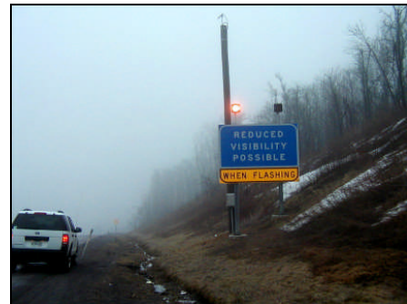
Figure 1. Typical “Reduced Visibility” Warning Sign
