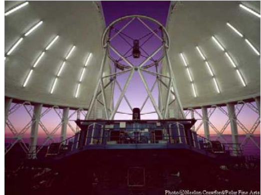
Gemini North dome/enclosure with setting sun (to left) lighting up bottom half of telescope through thermal vents (fully open). The observing slit is partially open revealing the truss and top end of the telescope. Credit: Gemini Observatory/AURA
