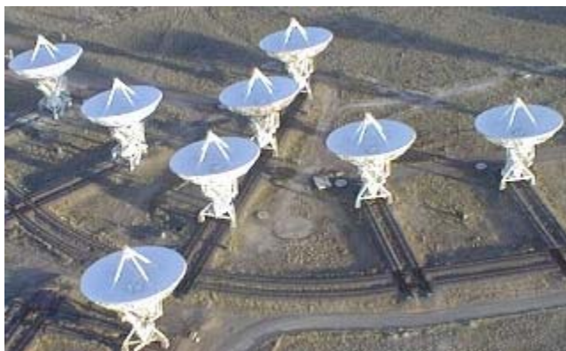
The Very Large Array, pictured here, consists of 27 radio antennas in a Y-shaped configuration on the Plains of San Agustin fifty miles west of Socorro, New Mexico. Each antenna is 25 meters (82 feet) in diameter. The data from the antennas is combined electronically to give the resolution of an antenna 36km (22 miles) across, with the sensitivity of a dish 130 meters (422 feet) in diameter.
