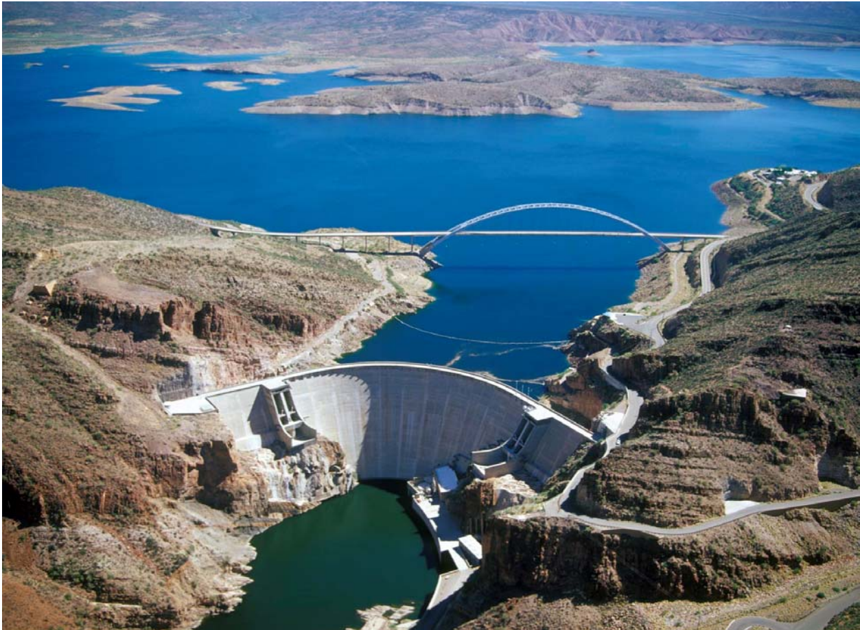
Figure 3. Roosevelt Dam in 1996 following modifications that raised the height of the dam 77 ft (23 m), increasing the storage capacity of the lake by roughly 20% (photograph by Reclamation).
