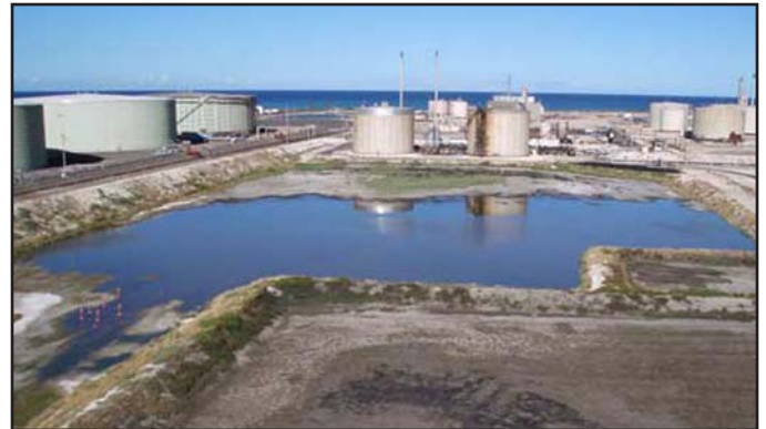
Rowlands Pond at Chevron Refinery. Photo courtesy of Jaap Eijzenga.
