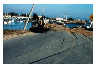
Loma Prieta, California, Earthquake 17 October 1989, Moss Landing. Damaged approach and abutment of the bridge linking the spit to the mainland. Liquefaction of the beach and Salinas River deposits caused ground cracking and differential settlement. Slide XV-2, USGS Open File Report 90-547 (<a href="http://130.11.57.28/of90547.htm">http://130.11.57.28/of90547.htm</a>), Digital File:tjc00009, ID. Tinsley, J.C. 9ct
