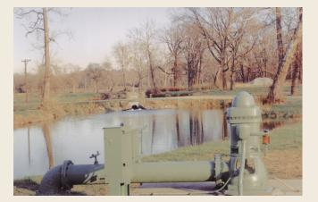
High-capacity turbine pump installed on a municipal well at Rohrers Island. Recharge lagoon in background. (Photograph by Brent Means, U.S. Geological Survey.)
