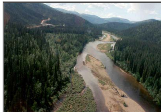
Upper Goodpaster River near 1525 Portal (at left)
