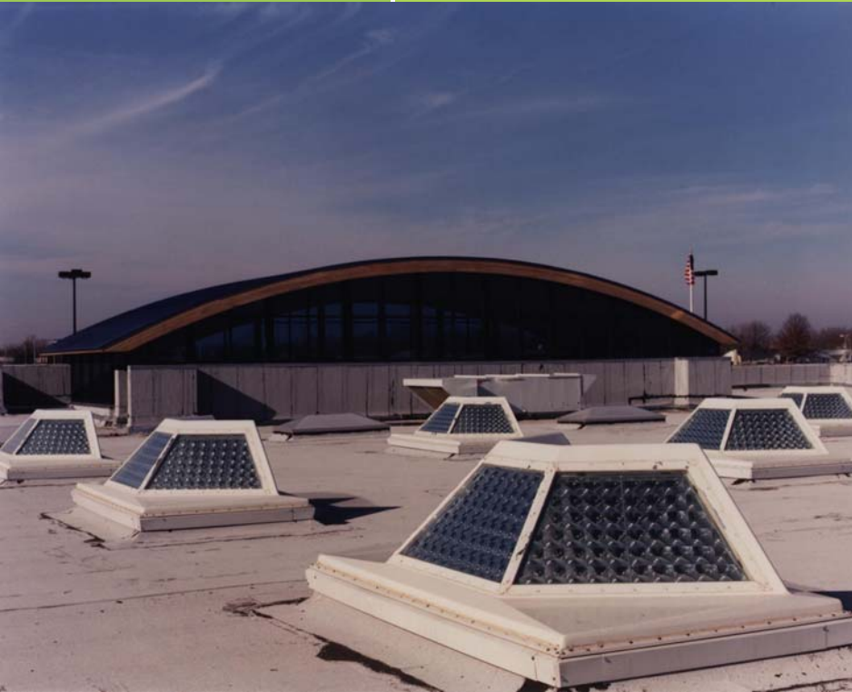
First generation of Anderson "Lighthouse" skylight used in Lawrence, KS
