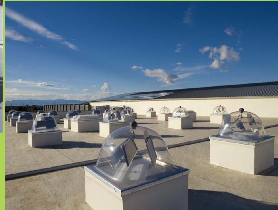
Current version of a solar tracking skylight test and evaluation in Aurora, CO-2006
