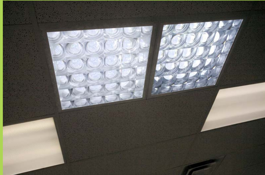
Current version of Solatube skylight used in Aurora, CO for use in offices and break rooms
