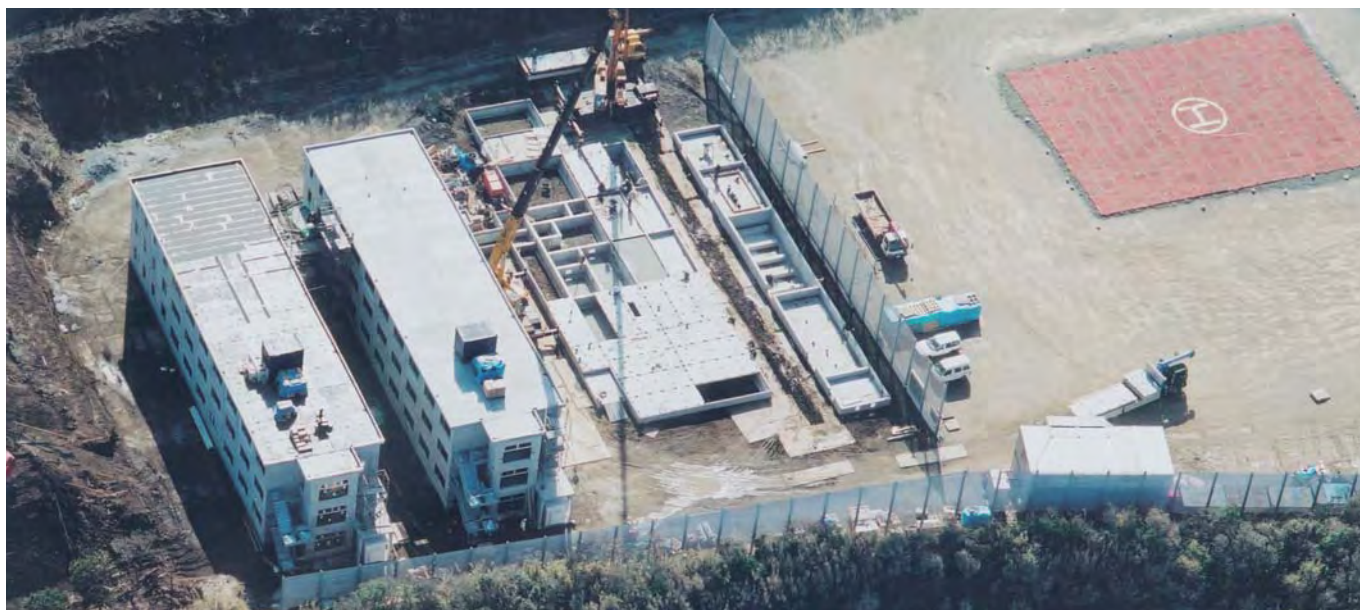
Izu Shelter under Construction
