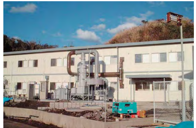
Desulphurization Equipment Installed in Accommodations
