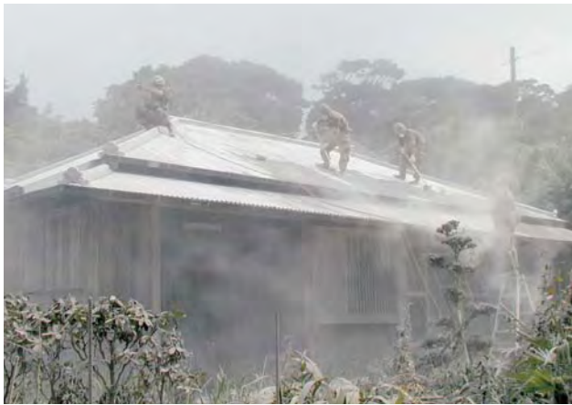
August 21: Self-Defense Forces Re-visit the Island to Remove Ash Accumulated on the Roads and Houses of the Elderly.
