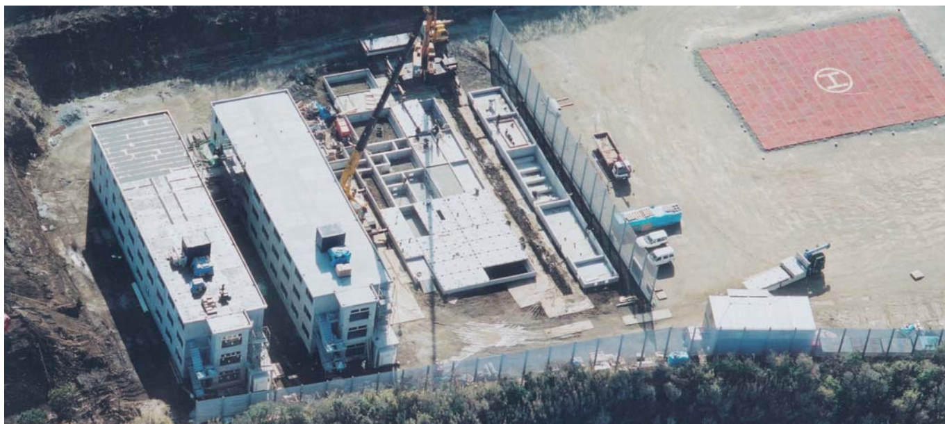
Izu Shelter under Construction
