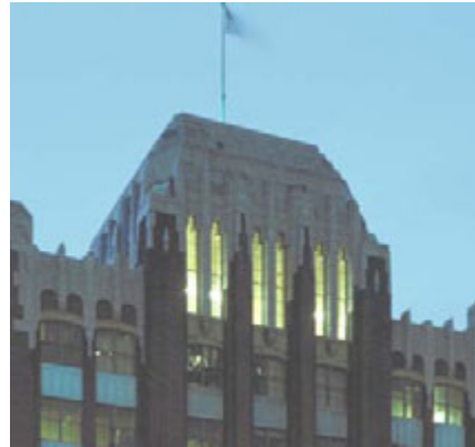
Federal office building, Seattle, Washington
