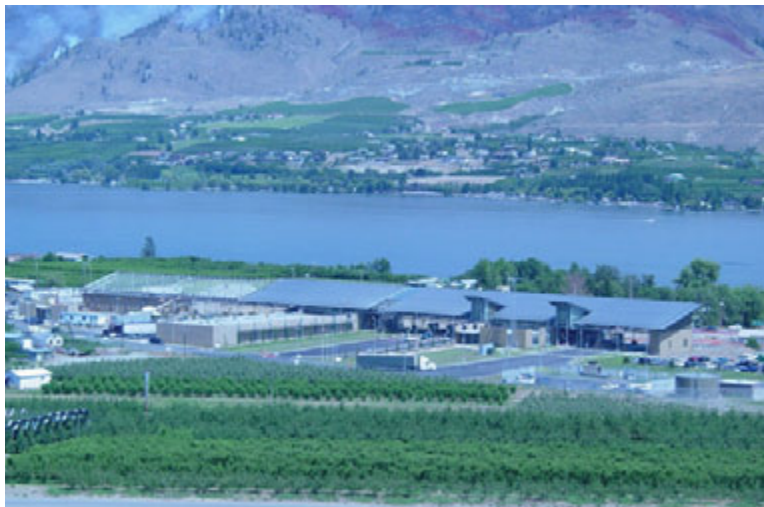
Planners incorporated sustainable features in the Border Crossing Station in Oroville, Washington
