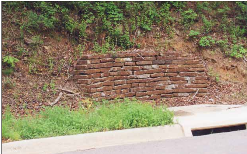
FIGURE 3 Curb/gutter and culvert with adjacent stone retaining wall.
