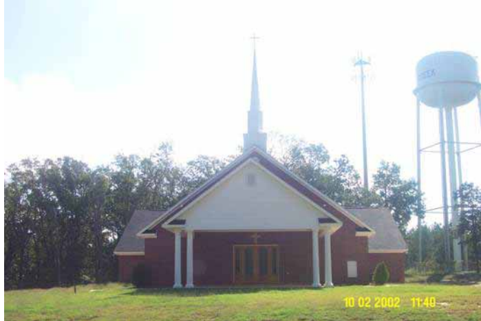
FIGURE 7 Consideration was given to properties important to the community, like this church.
