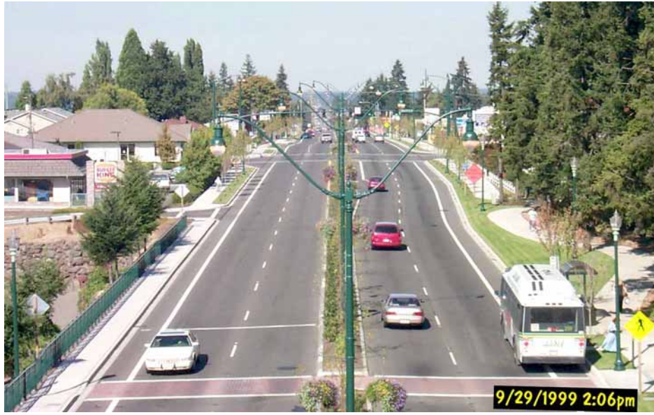
FIGURE 3 Bridgeport Way after, north view.
