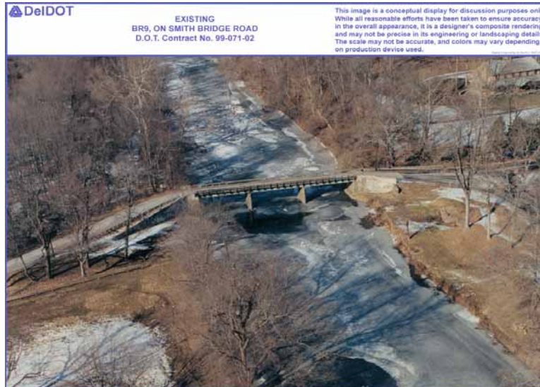
FIGURE 1 Existing bridge structure.
