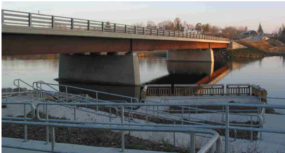
FIGURE 4 Completed Salmon River Bridges.
