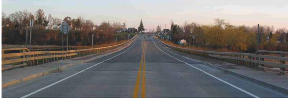
FIGURE 3 Salmon River Bridge (looking south).
