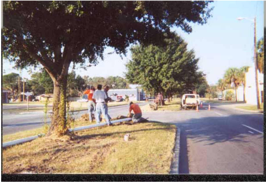
FIGURE 7 Martin Luther King Boulevard median construction.
