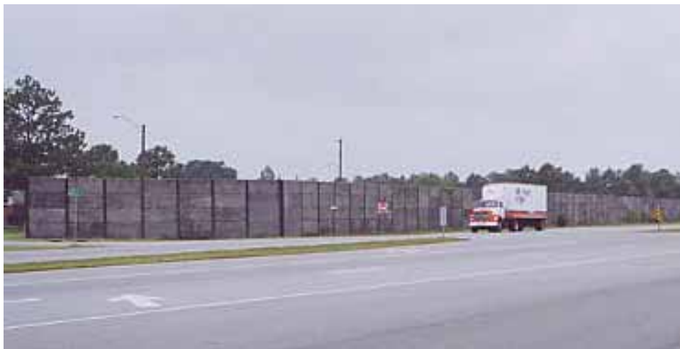
FIGURE 4 Noise walls in Section C.
