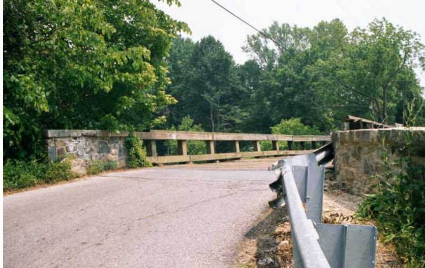
FIGURE 2 Existing west side of bridge.
