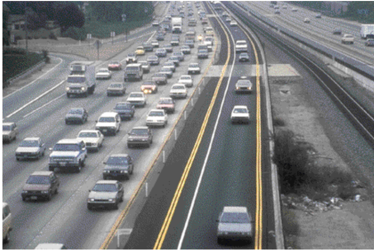
Figure 3. El Monte Busway Buffer Separated Section
