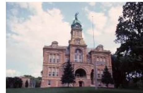
Blue Earth County Courthouse Mankato, MN
