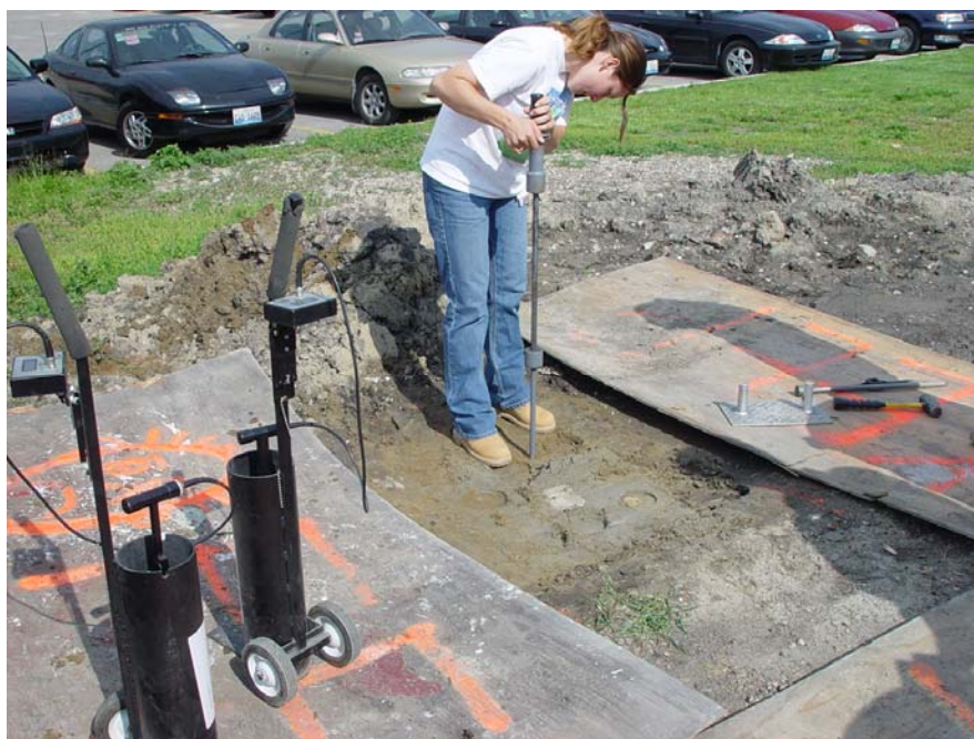
Figure 17 – Utility DCP test on the soil during forensic study
