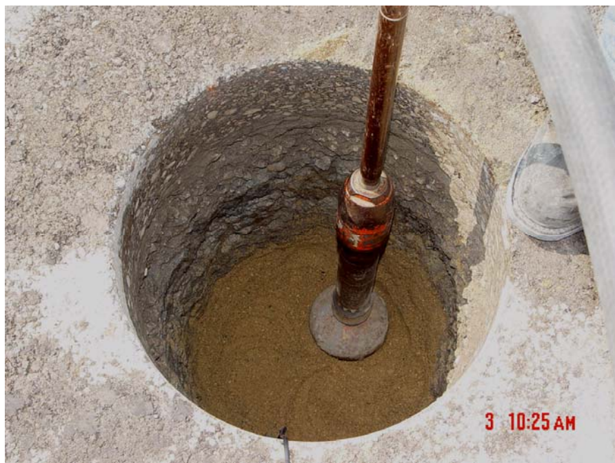
Figure 12 – Compaction of the keyhole section
