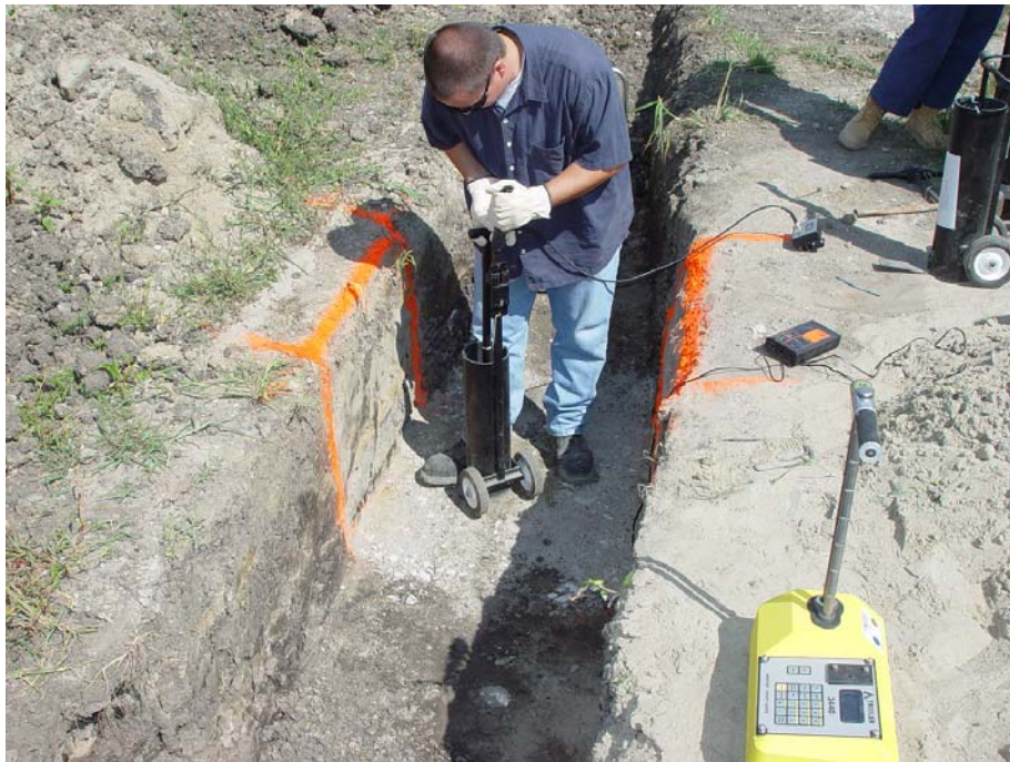
Figure 57 – Use of the Clegg Hammer to evaluate compaction in trench backfill
