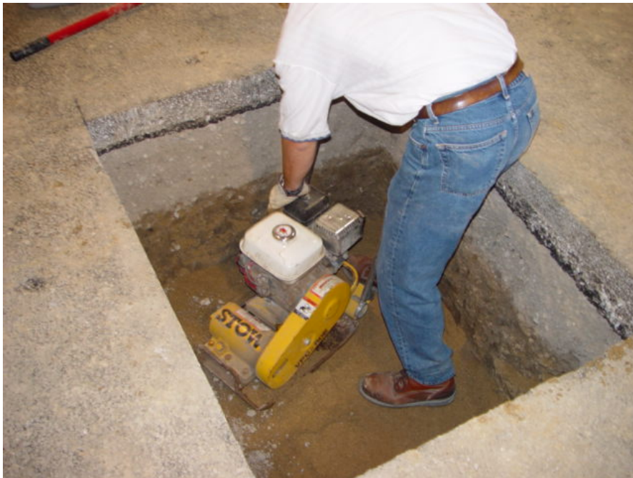
Figure 6 – Compaction of sand using vibrating plate in the bellhole
