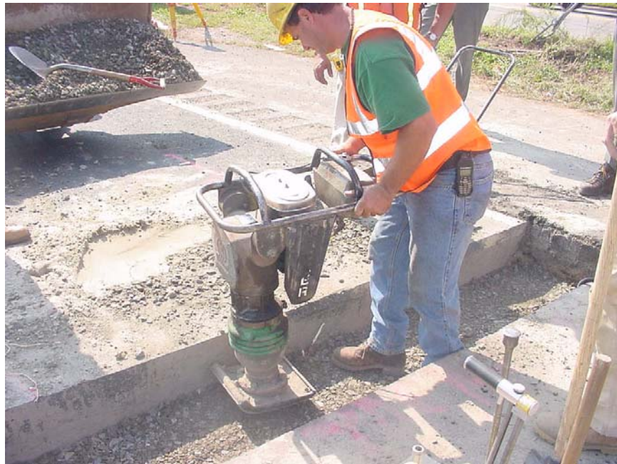
Figure 23- Compaction of the 20-inch wide trench in the NJ site
