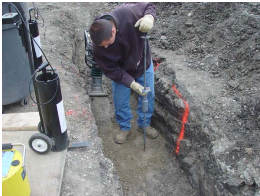
Figure 19 – Using the Utility DCP in the silty-clay trench
