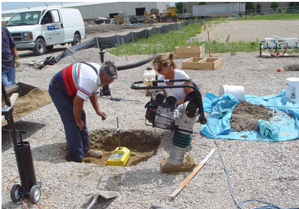
Figure 21 – Density measurements of the outdoor bellholes using the NDG
