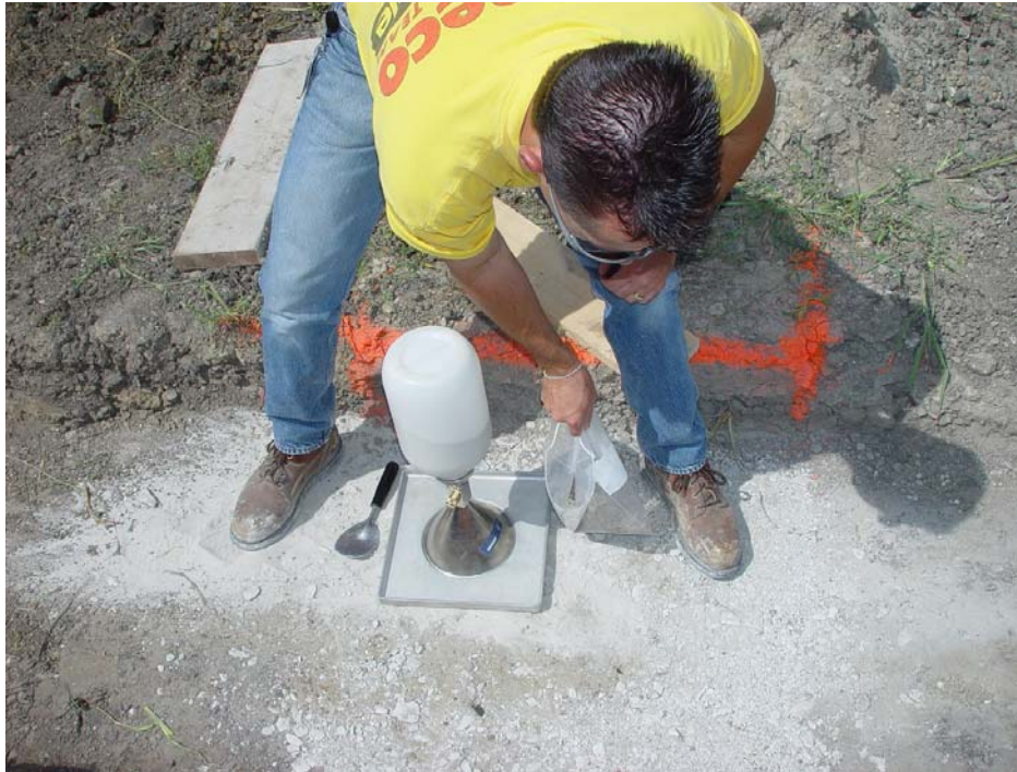
Figure 34 – Use of the sand-cone apparatus in the stone-base trench
