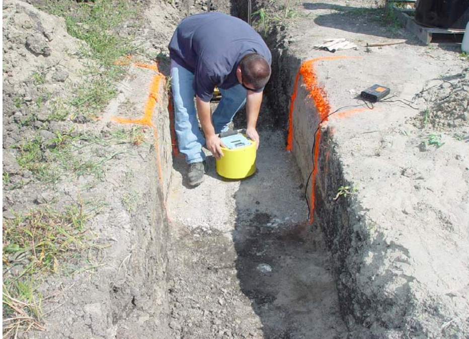
Figure 49 - Use of the Geogauge to evaluate compaction in trench backfill
