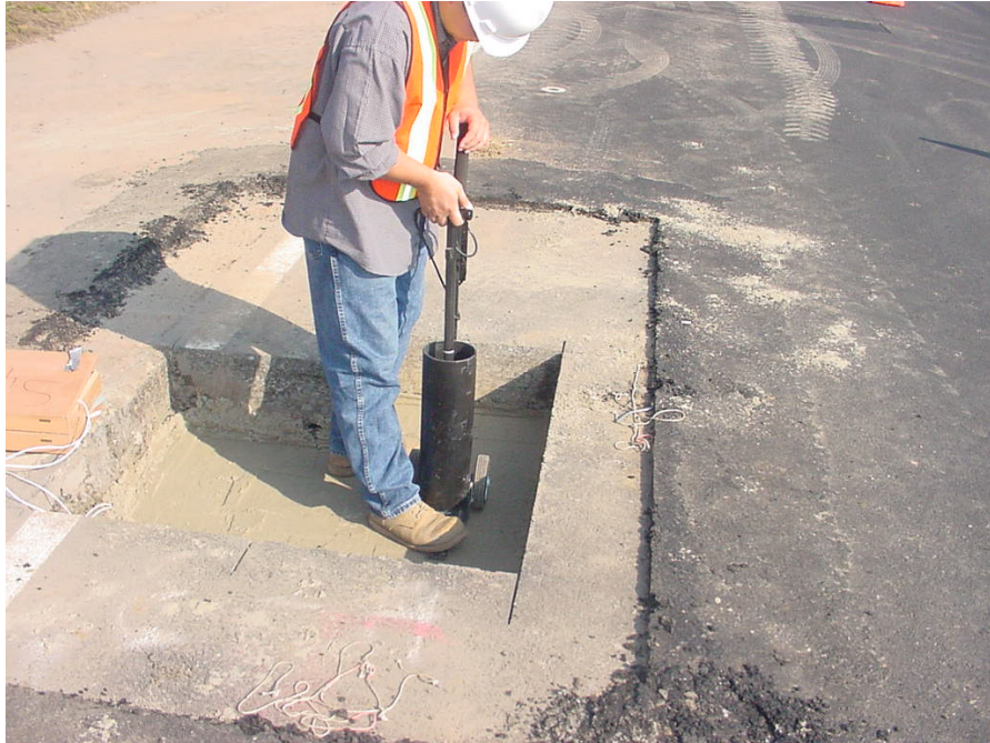
Figure 22- Compaction measurement of the bellhole using the Clegg Hammer
