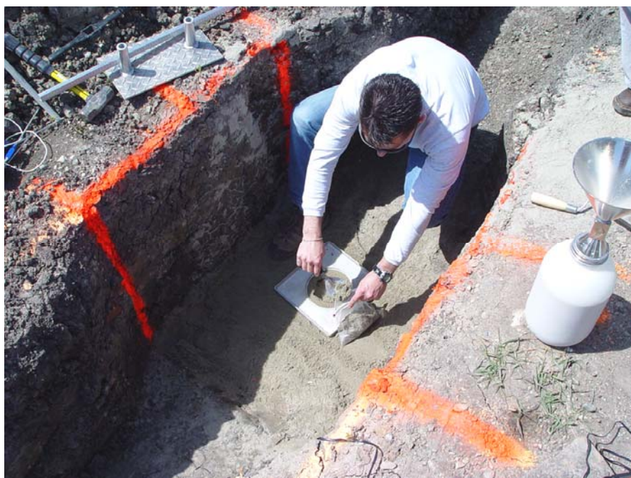
Figure 16 – Sand-cone test on the NJ-Sand trench
