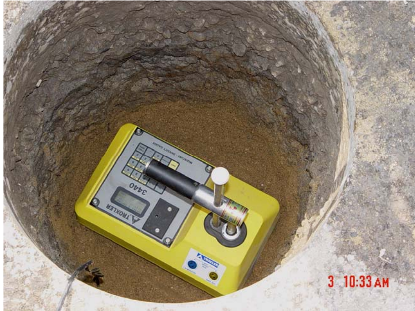
Figure 13 – Compaction measurements in the keyhole using the NDG
