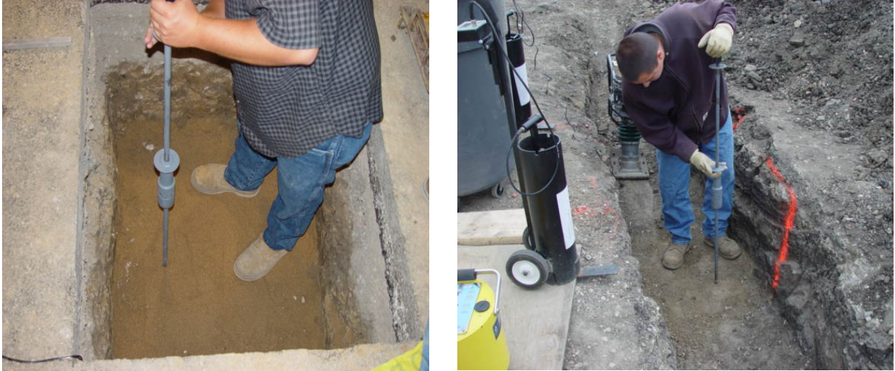
Figure 41 – Use of the Utility-DCP in bellhole and trench backfills
