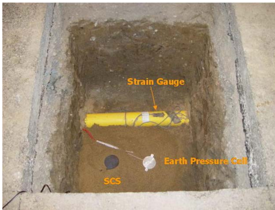
Figure 4 - Bellhole test section Sand-1
