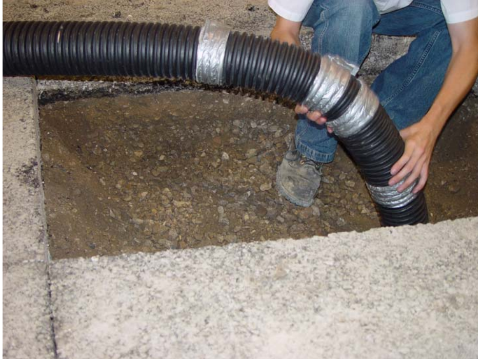
Figure 7 – Vacuum excavation of the compacted backfill
