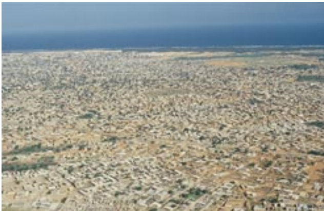
Aerial view of Pikine in the suburb of Dakar. Although Pikine was created just 20 years ago with the objective of alleviating congestion of the Senegalese capital, Dakar, it has rapidly grown to a city of more than 800,000 inhabitants. A poor rural economy and drought have increased the rural to urban migration, contributing to Pikine's rapid growth. Its density exceeds 10,322 inhabitants per km 2 .
