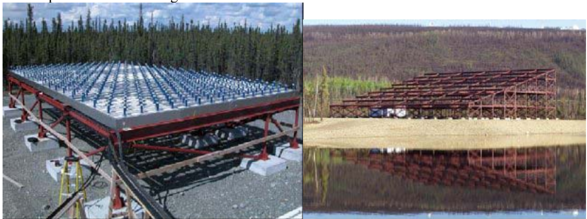
The left view shows the 16 panel installation of AMISR units at Gakona, Alaska. The right view shows the frame for the installation of a complete AMISR face at Poker Flat that will be completed during Fall 2005 and Spring 2006.
