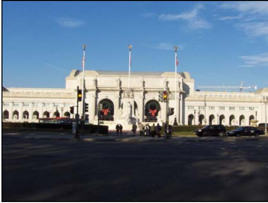
Fig. 2 – view north through Columbus Plaza toward center portico and flanking loggias on south (front) elevation of Washington Union Station.
