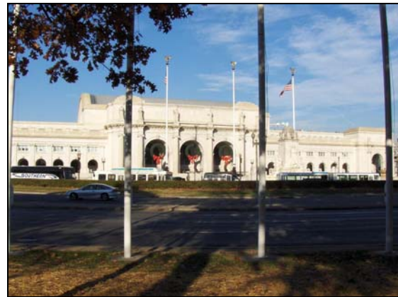
Fig. 3.3 – general view looking north through the state and territory flags, and through Columbus Plaza toward the front of the station. Even without the tour buses, note how the topography of the Plaza will reduce the visual impact of the proposed bollards.
