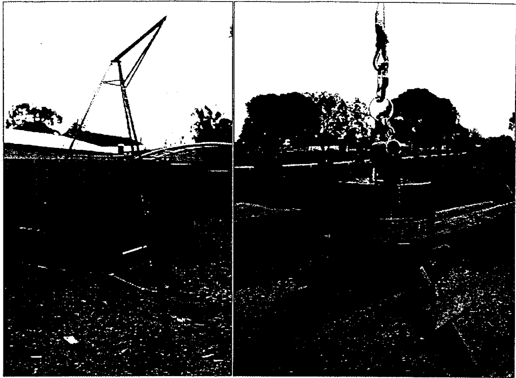
Figure 47: Drop rig and head form used to determine compliance of ground surface shown in Figure 48.
