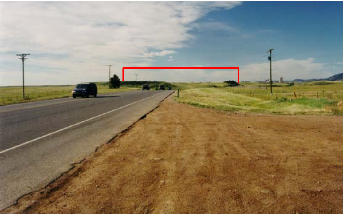
1. View of the NWTC looking south from the shoulder of Highway 93 on June 25, 2001.
