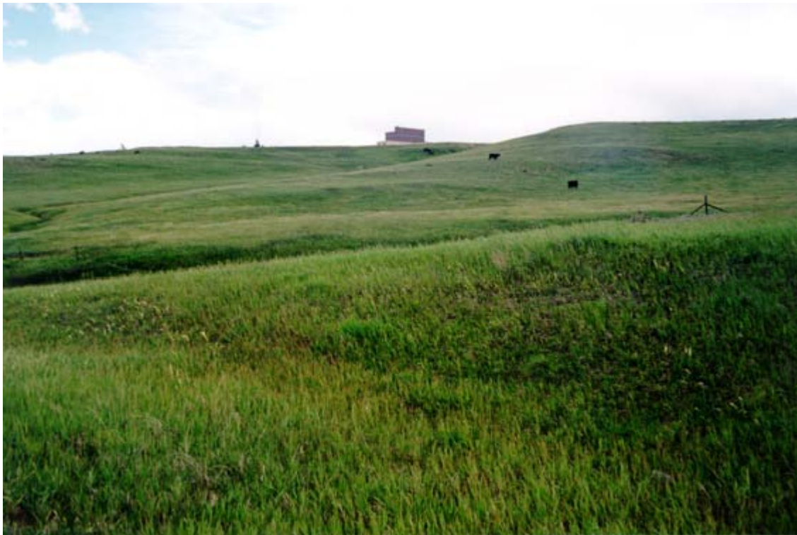
12. View of Building 251 from Highway 128 north of the project site access road.
