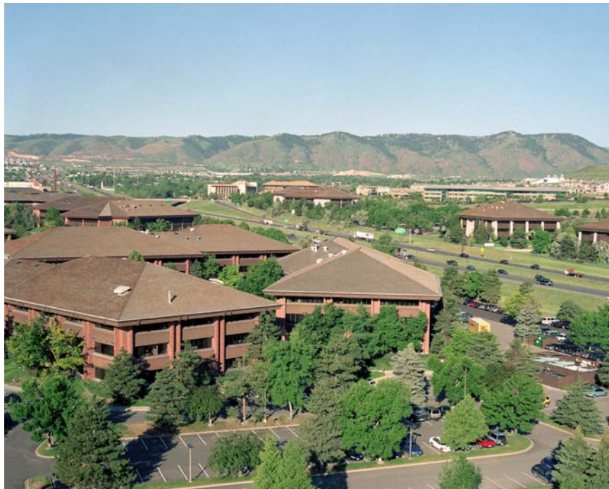
Figure 1.8. South Table Mountain Site – Denver West Office Park.
