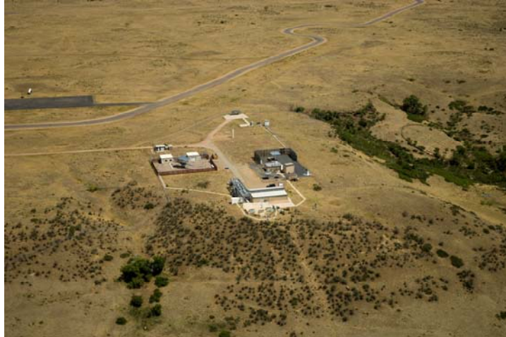
Figure 6.2. STM Site easement lands.
