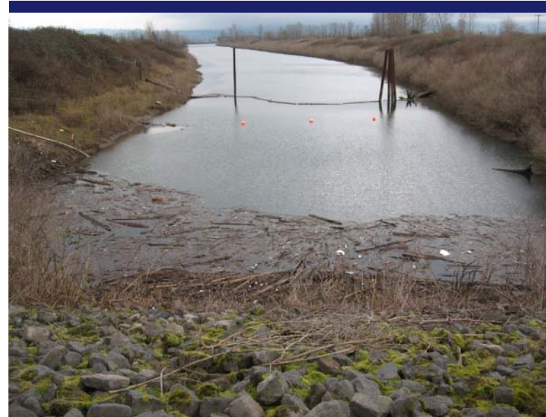
Photo 6 Flushing Channel inlet.
