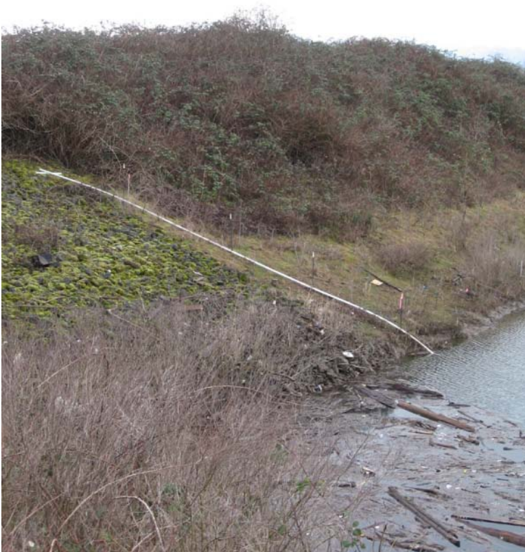
Photo 7 Pipe of unknown use.
