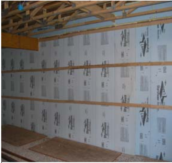
Figure 13. Foundation insulation with furring strips
