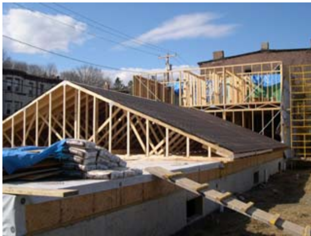
Figure 8. Two roofs with sheathing and tarpaper — ready for the crane
