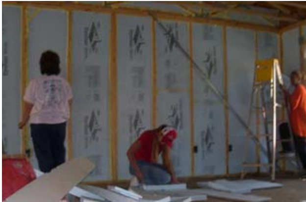
Figure 15. Volunteers cut insulation to fit in above-grade walls
