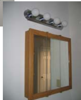
Figure 23. Strip light with CFLs
