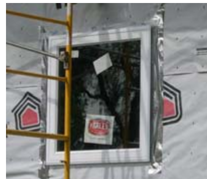
Figure 11. Window installed and flashed
