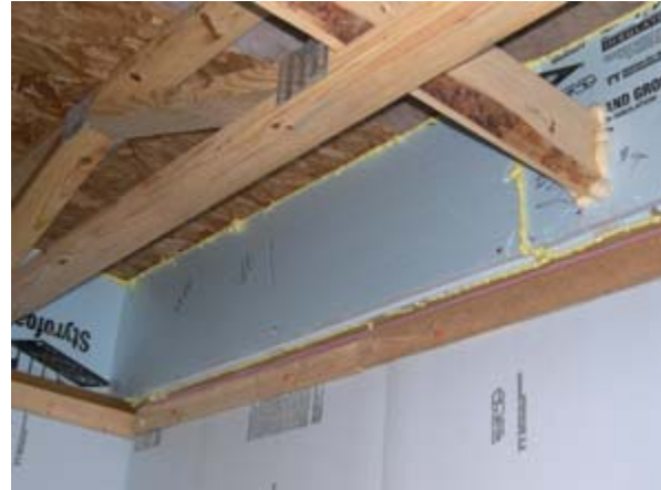
Figure 14. Band joist insulation cut to fit and sealed with foam
