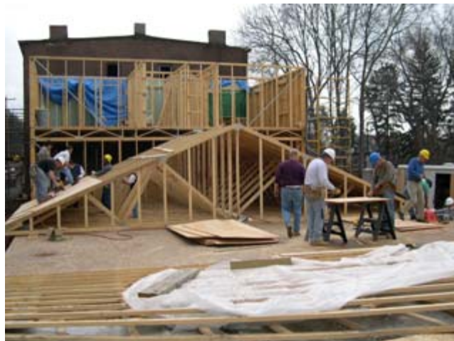
Figure 7. Building each roof on the deck of the next unit
