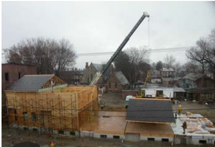
Figure 9. Lifting the roofs into position
