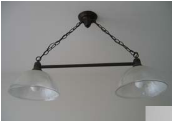
Figure 21. Chandelier with two 15-Watt CFLs
