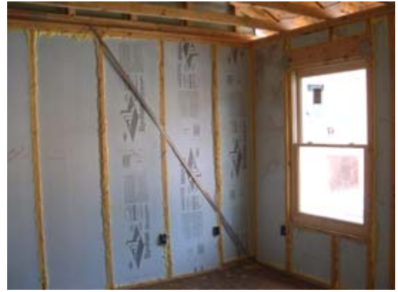
Figure 16. Finished wall with foam around each piece
