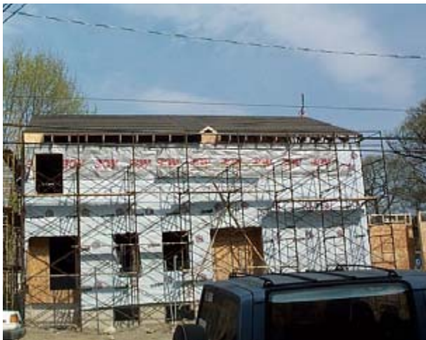
Figure 10. First two roofs in place
