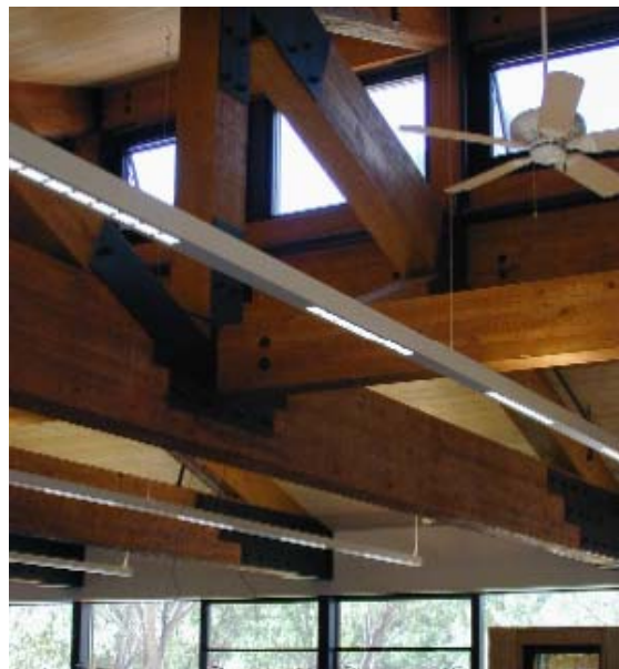
Figure 3-16 Zion's 88% uplighting with T-8 fixtures (note the dark ceilings and beams combined with minimal down lighting)
