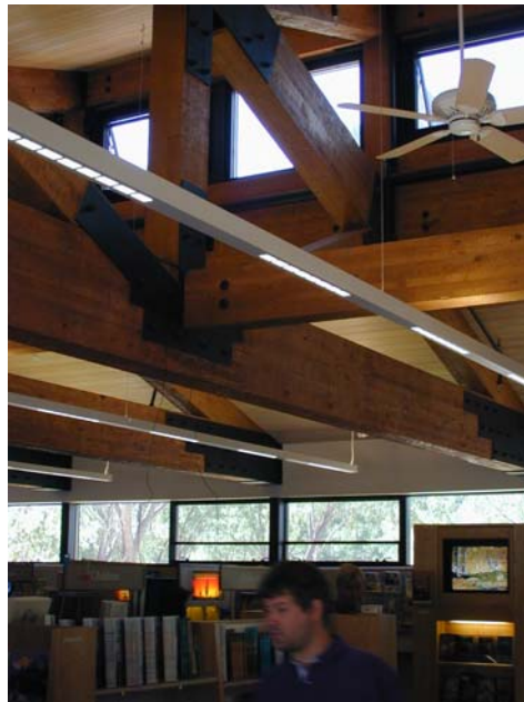
Figure 3-8 Zion daylighting with fixtures that are 88% indirect and 11% direct
