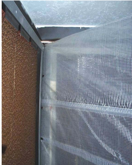
Figure 3-31 Plastic blocking device for cooltowers
