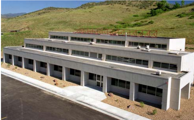
Figure 3-4 TTF daylighting with clerestory
