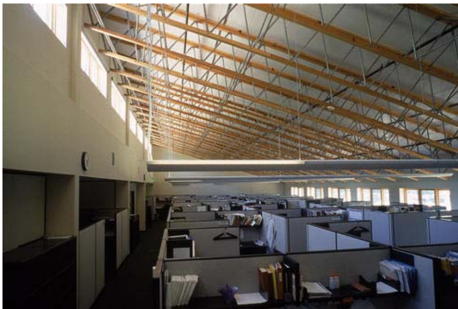
Figure 3-7 Cambria second floor clerestory showing dark floors and high vaulted white ceilings with an open truss
