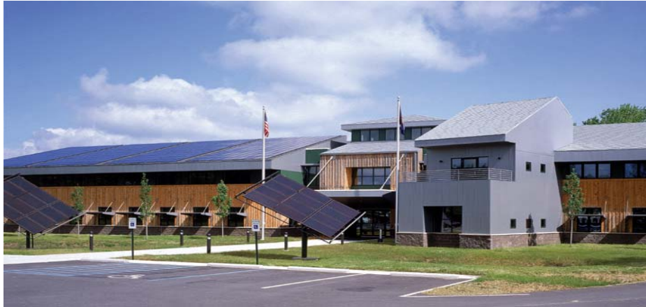
Figure 2-3 South elevation of the Cambria Office Building
