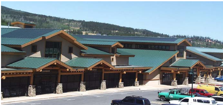
Figure 2-6 BigHorn Home Improvement Center
