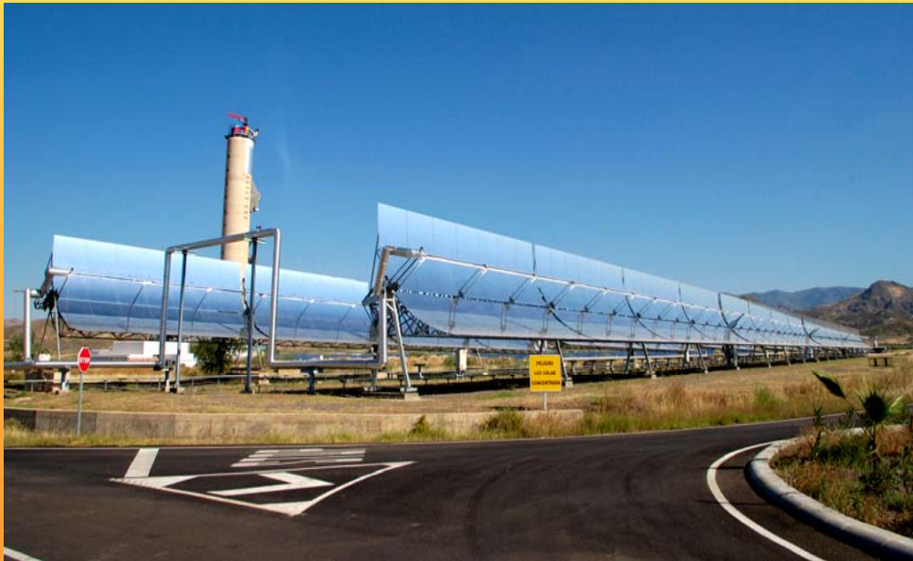
The DISS solar field (south)
