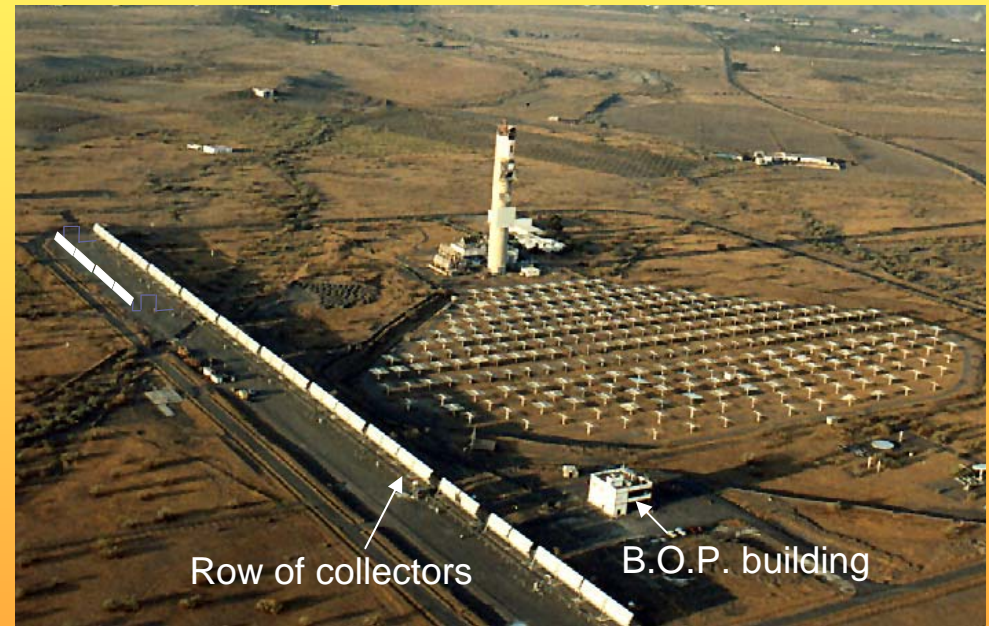
Aerial view of the DISS facility
