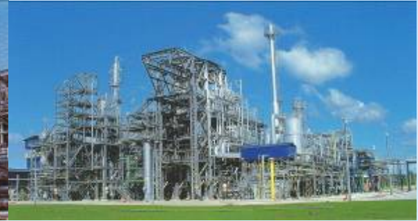
b) Molten Salt system with an output of 7.7 MW at 470°C, melamine plant in Germany
