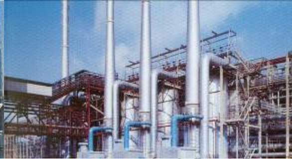
b) Molten Salt system with an output of 88 MW at 400°C, Bauxite digestion plant in Germany
