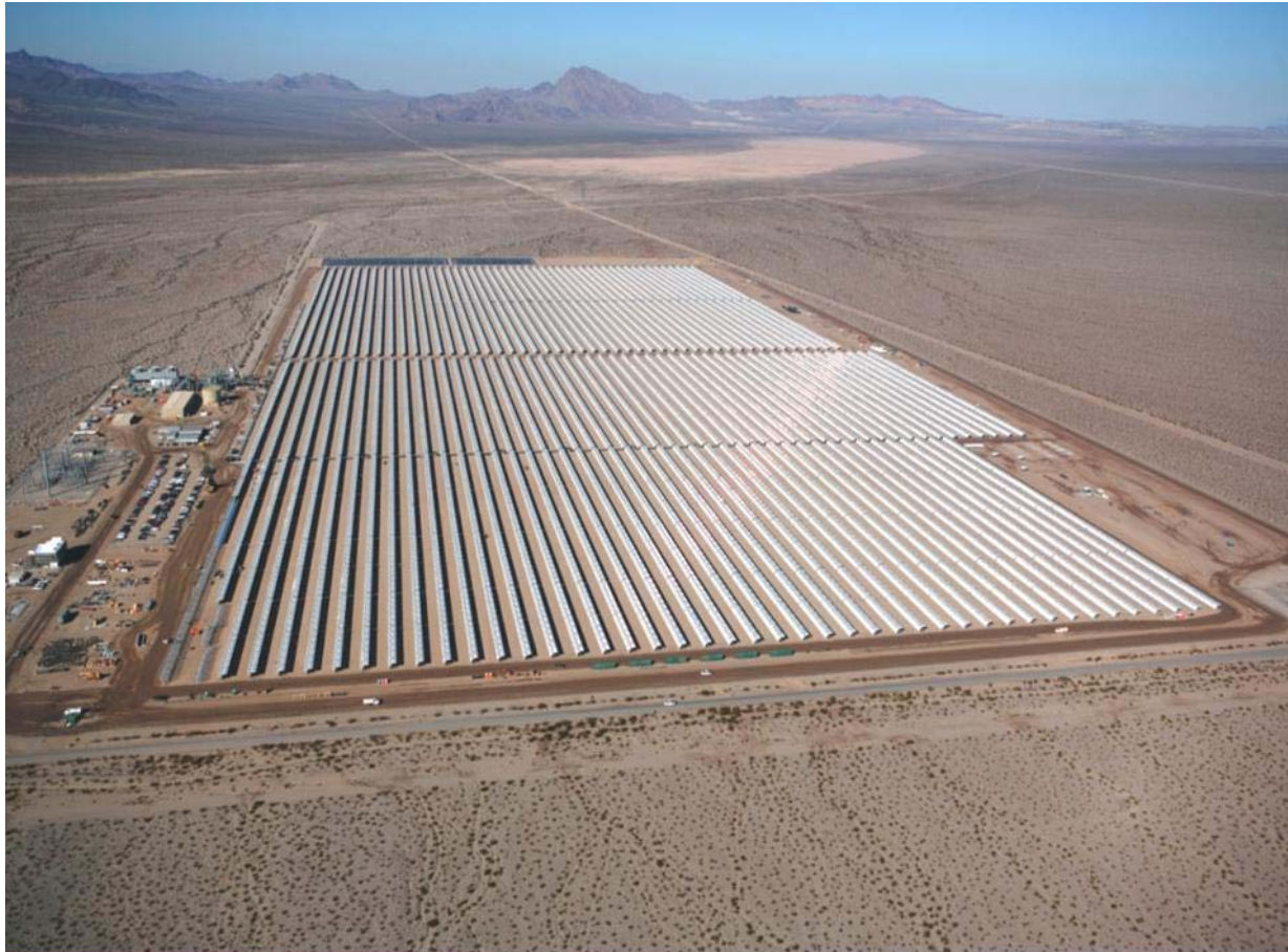
NEVADA SOLAR ONE - ACCIONA SOLAR POWER - 64 MW - Boulder City, NV
