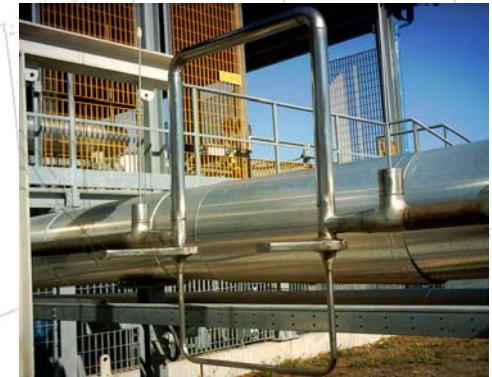
Special equipment for piping operation
