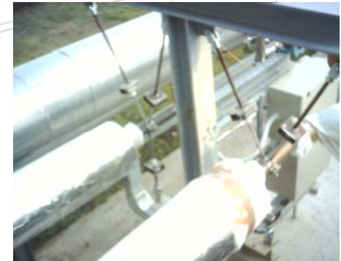
Electrical/thermal insulated hangers for Joule effect direct heated piping
