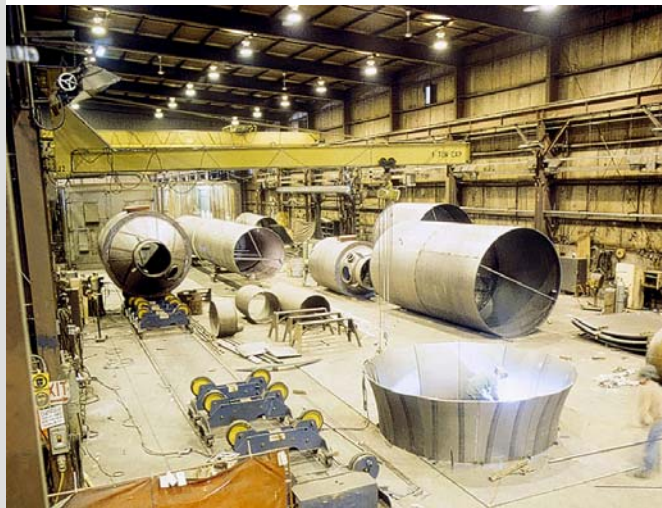
Courtesy of Caldwell Energy Division Of Caldwell Tanks, Inc.
