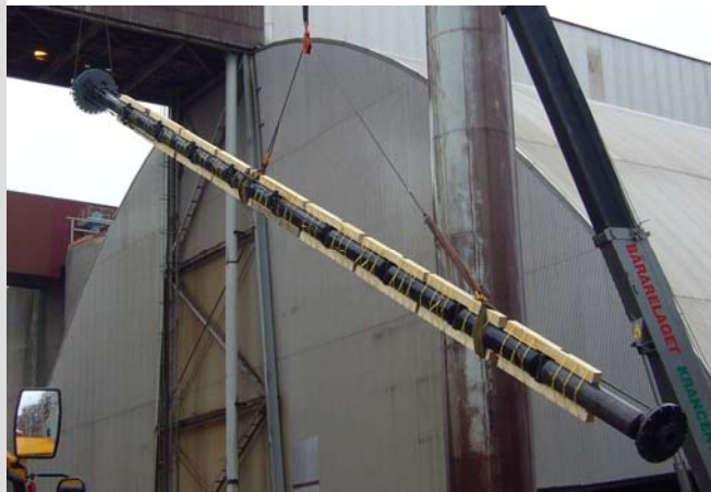
Above is a 17 Meter long High Temperature pump Molten Sulfur
