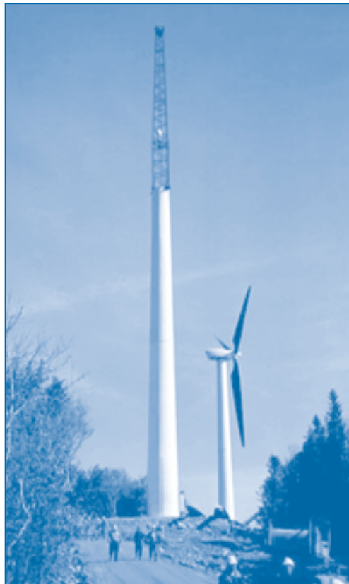
Wind Farm Under Construction
