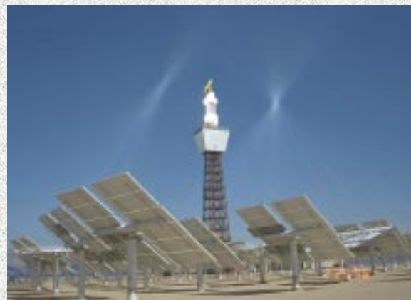
Solar Two at Daggett, California
