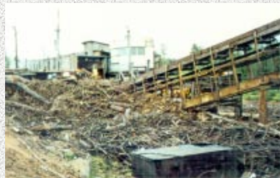
Site for a 1-MW Biomass Power Plant in Verkhne-Ozerski village, Arkhangelsk Region that will burn nearby wood waste.
