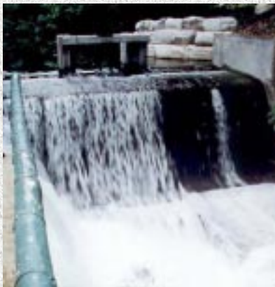
A view of the micro-hydro plant
