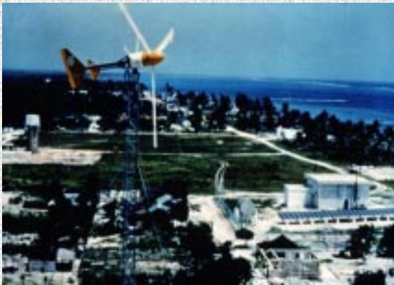
Xcalak hybrid power system - diesel retrofit completed in 1995
