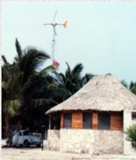
Costa de Cocos 11-kW wind-diesel hybrid system
