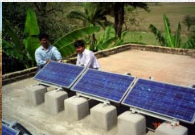
PV modules generally range in size from 50 W to 130 W and can be installed by one to two people. Several modules can be interconnected for more power.
