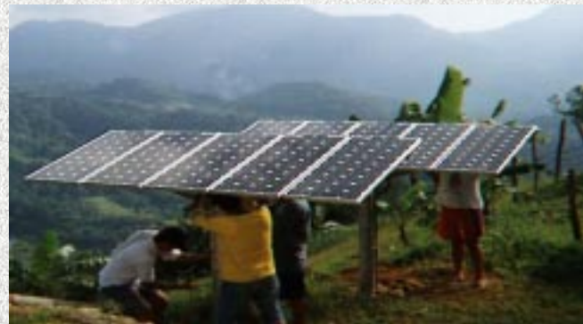
Panels installed by Solar Electric Company generate electricity to power a radio repeater station at the Regional Health Center of the Department of Health in Ormoc, Leyte
