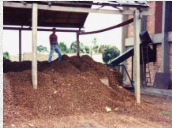
Riberalta biomass 1-MW power plant
