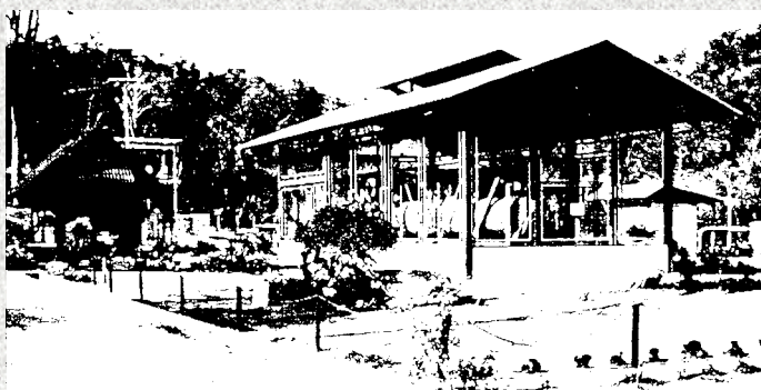
A 300-kW geothermal binary plant has operated for four years in Fang, Thailand.
