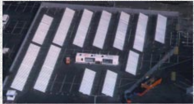
Aerial view of a CAN! facility near the Los Angeles airport
