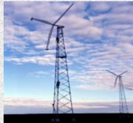
50-kW turbines in Kotzebue, Alaska
