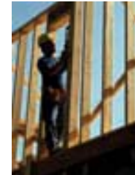
New Homes Construction
