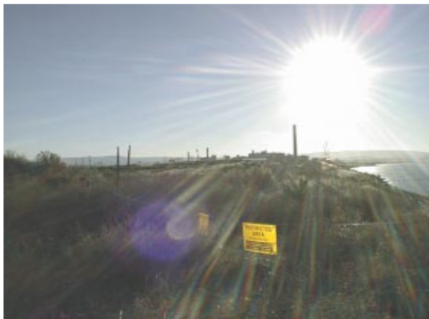
Hanford “N” Reactor Adjacent to the Columbia River (Source: Phil Weihrouch, EPA OIG)
