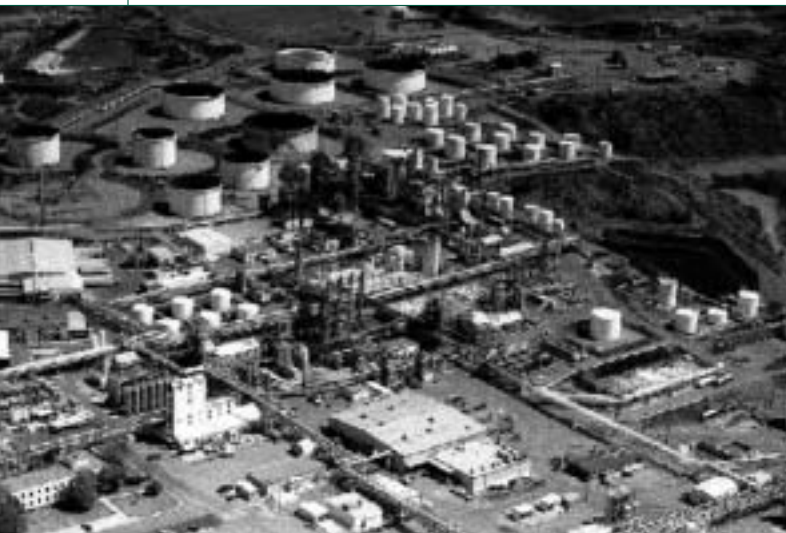
The DECSE fuels were blended at the Chevron Phillips Chemical Company, LP, in Borger, TX.
