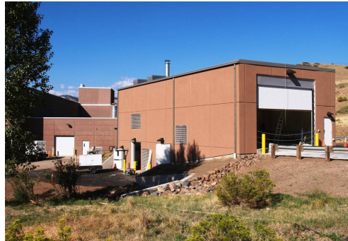
The Renewable Fuel Heating Plant will use urban wood wastes from Colorado's Front Range for fuel.
