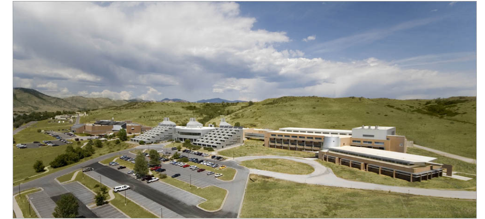
The Laboratory's permanent site near South Table Mountain will soon expand with the addition of an administrative support building, wood-fired boiler plant and more.
