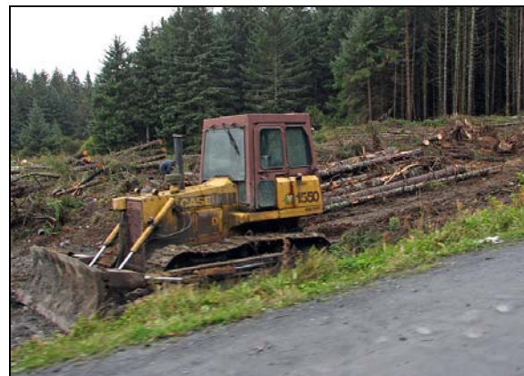
Clearing Trees for Fence Around Dump
