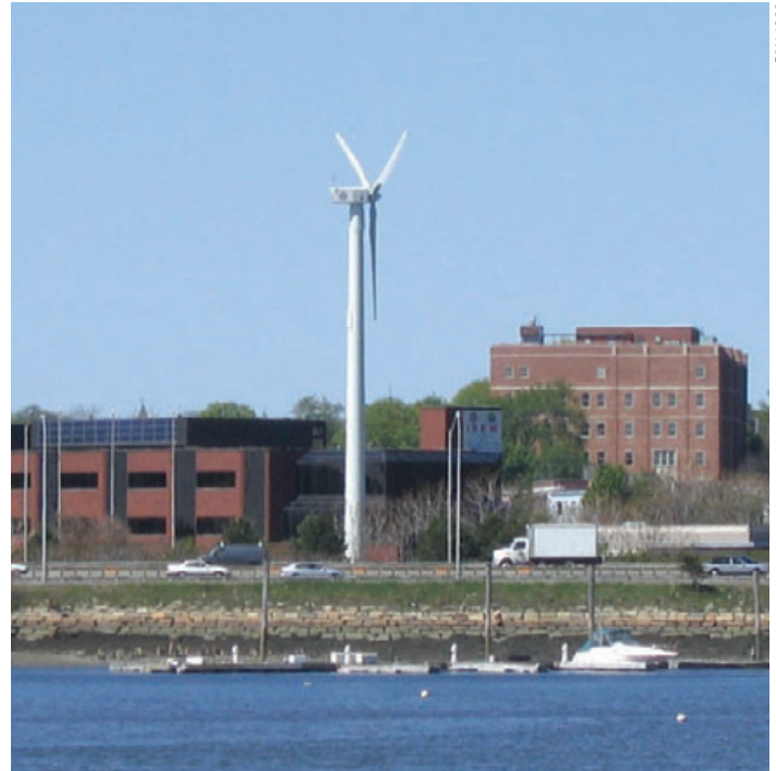
Fuhrlander FL100 wind turbine at the IBEW Local 103 headquarters, Dorchester, MA (courtesy IBEW Local 103)
