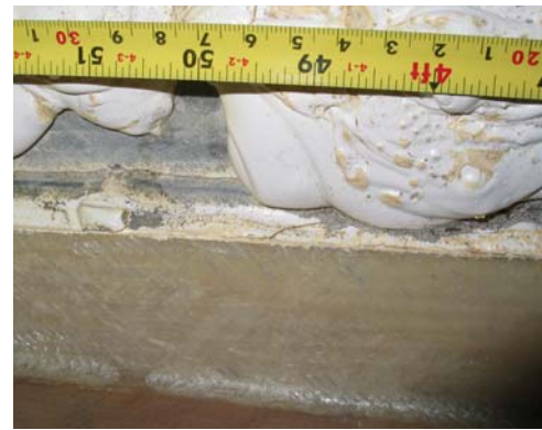
Figure 23: Crack in shear web to LP skin bond joint at 1.20-1.30 m on the CX-100 blade.
