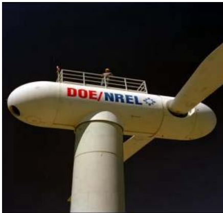
Figure 1. The Controls Advanced Research Turbine (CART).
