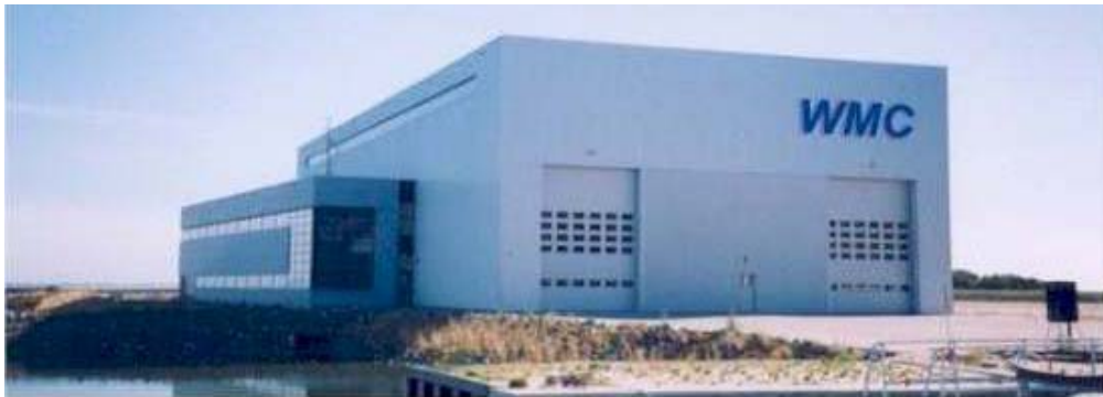
Figure 11: The WMC blade test facility
